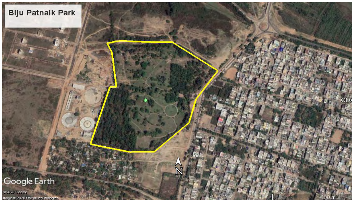
Figure 11: RWH structures in Biju Patnaik Park, Cuttack
