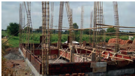
Bamboo reinforced concrete
