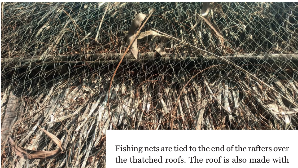
Fishing nets, tied over roof structures
