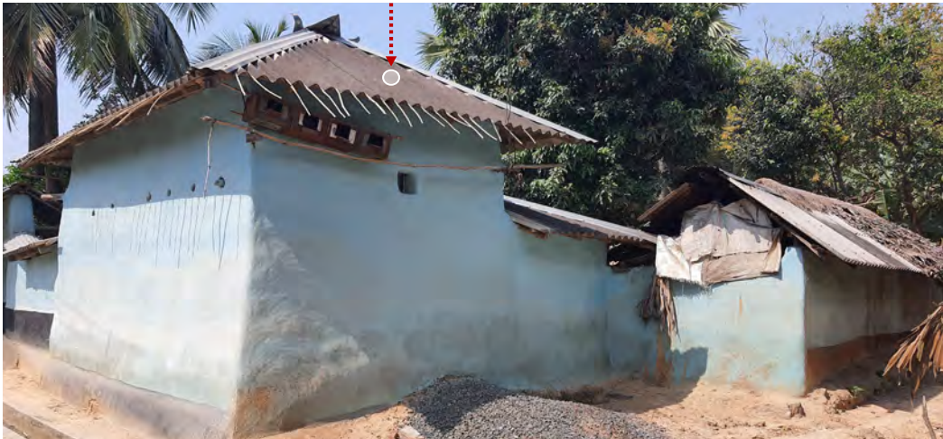
Asbestos roofing
