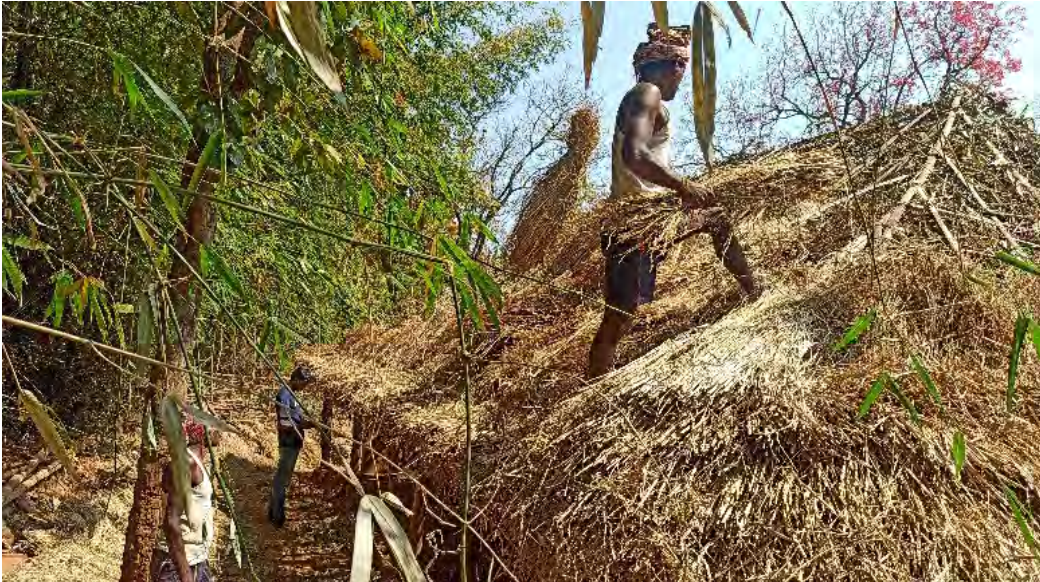
One worker on the ground passes the thatch bundles to another worker on top
