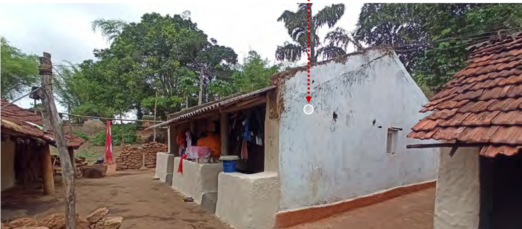
Cement plaster over brick wall
