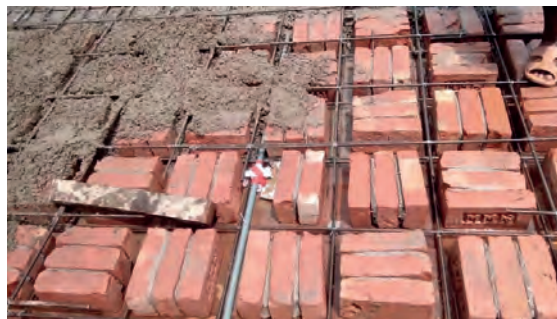
Reinforced Brick Concrete (RBC) slabs
