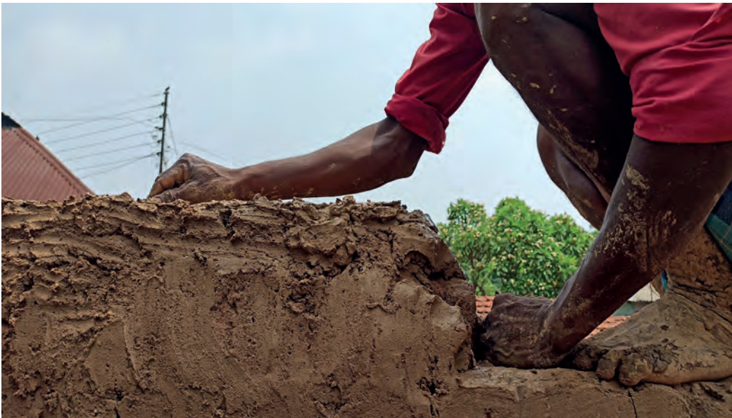
Evenly spreading and shaping the soil mound using hand
