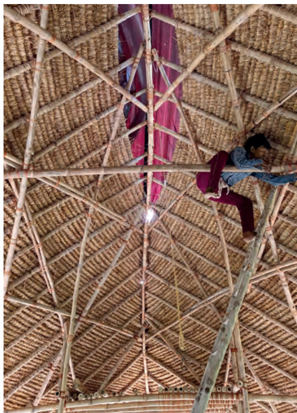
Roof made from bamboo and rice thatch
