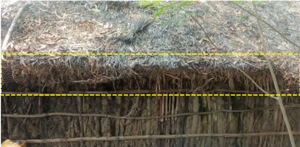
Thatched roof with fishing nets layered over it
