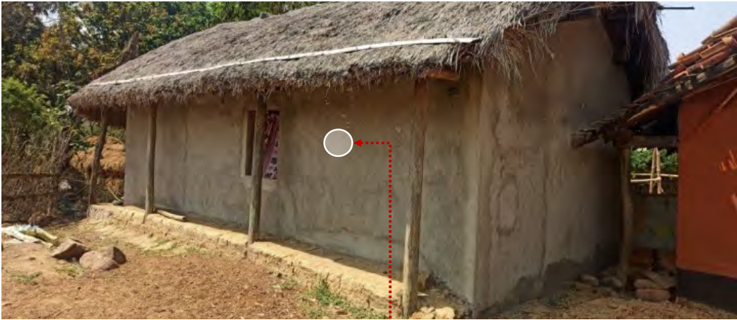
Cement plaster over brick walls
