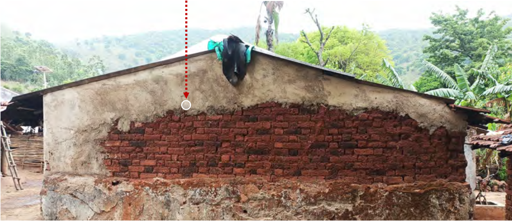
Red bricks and mud mortar
