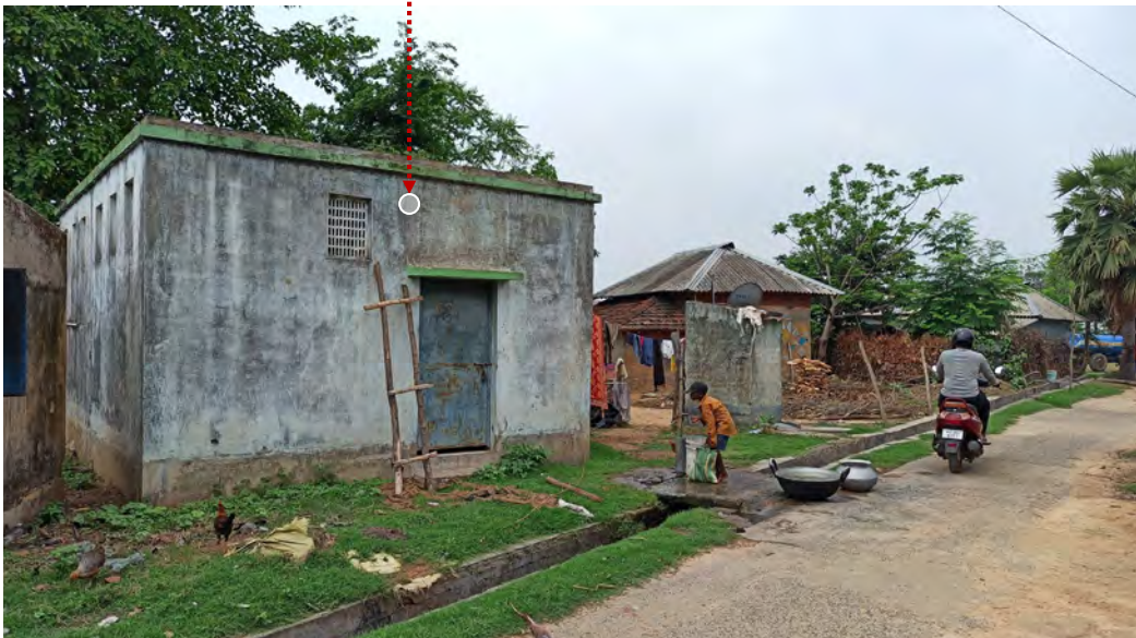
Brick and cement mortar
