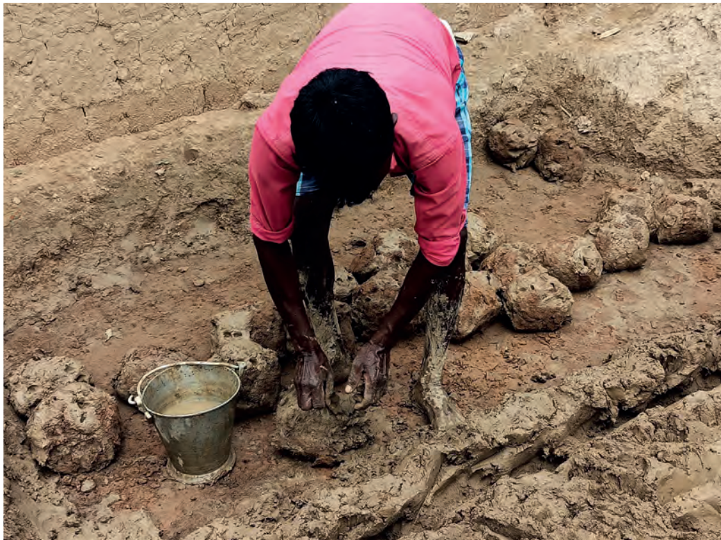
Maintaining the semi-clayey state of the lumps by sprinkling water
