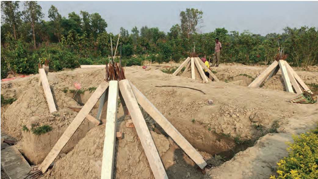
Chicken mesh layer, used for making the reinforcement for staircases.
