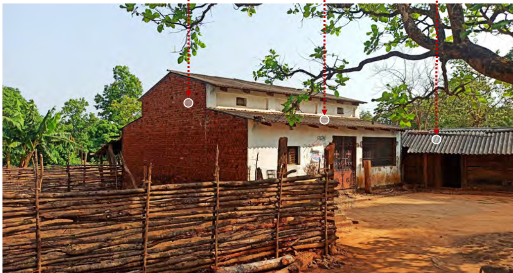
Asbestos roofing
