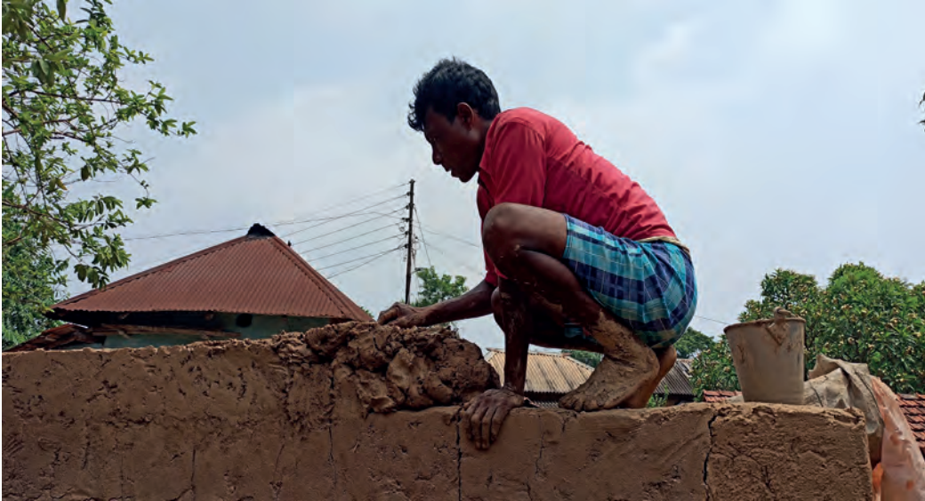
Placing of soil lumps onto the wall
