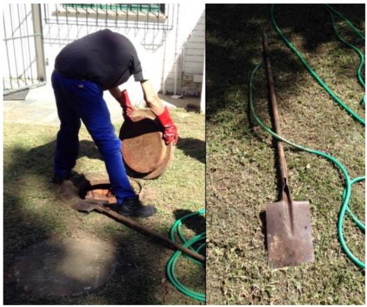
Opening the first compartment of septic tank
