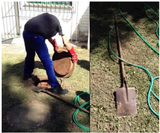
Opening the first compartment of a septic tank
