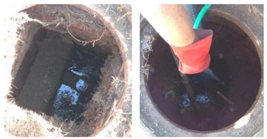
In Iact invert level in the second chamber and watering down to loosen the sludge
