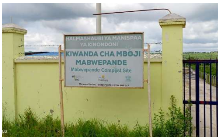
Entrance to the Mabwepande Compost Site owned by the Kinondoni Municipal Council
