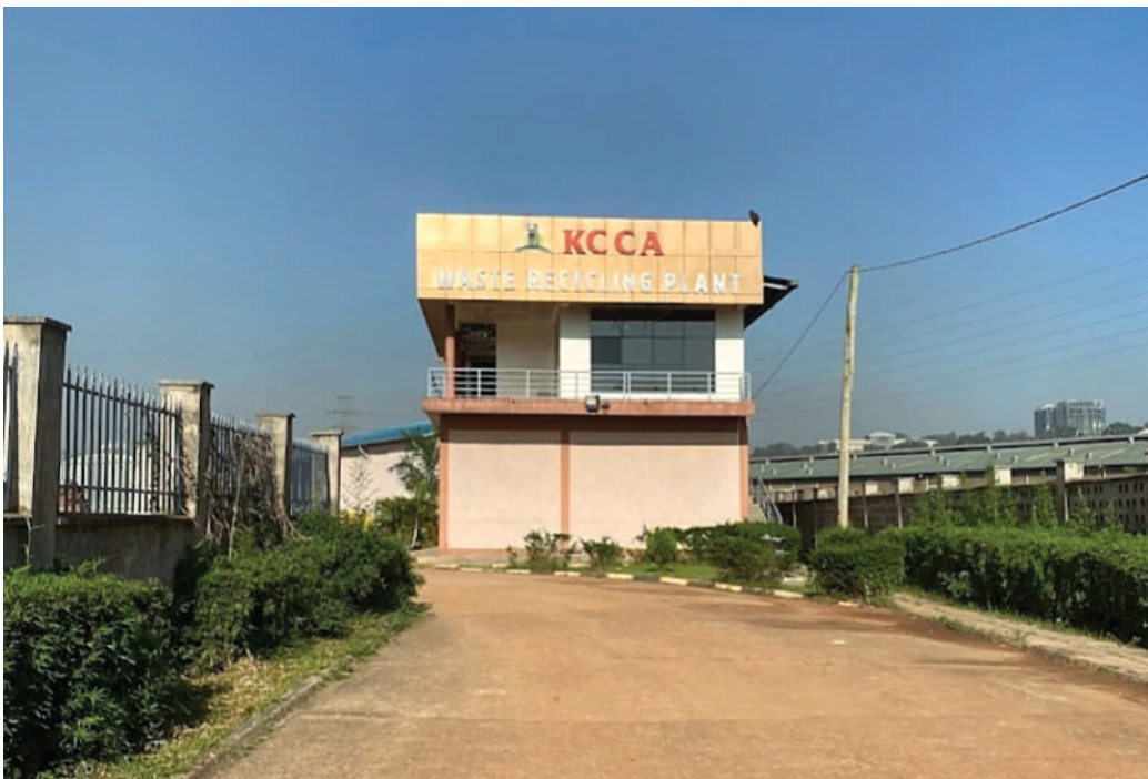
KCCA Waste Recycling Plant in Wankoko
