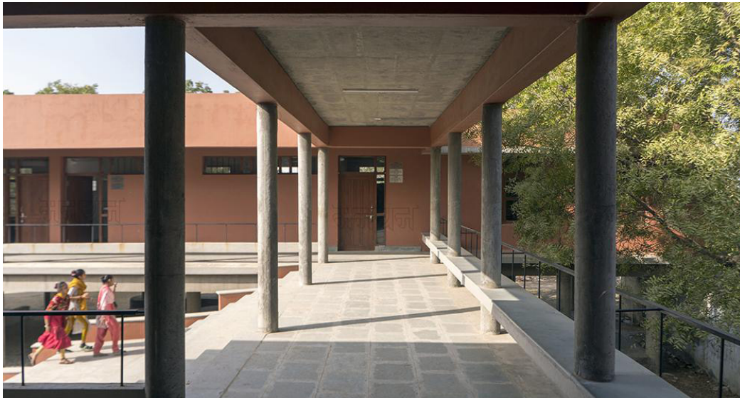
Courtyard planning that facilitates ventilation and mutual shading in Mahatma Gandhi Education Trust School in Mandal, Gujarat
