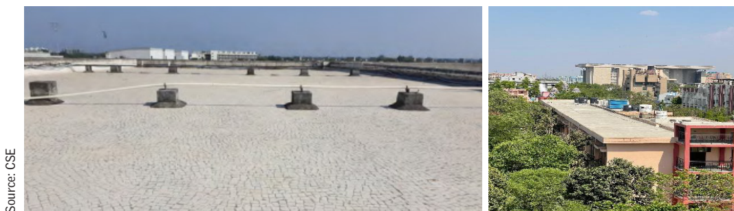
Cool roof strategy using white tiles (left) and reflective paint (right)
