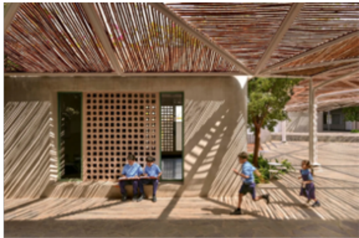
Sun shade constructed from bamboo for open spaces in Penna Foundation School, Talaricheruvu, Andhra Pradesh
