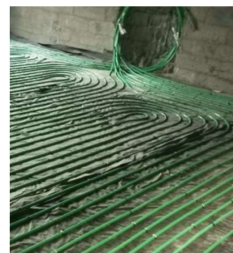
Image: Structural cooling being installed in Government Sarvodaya Co-Ed School in Mehram Nagar, New Delhi
