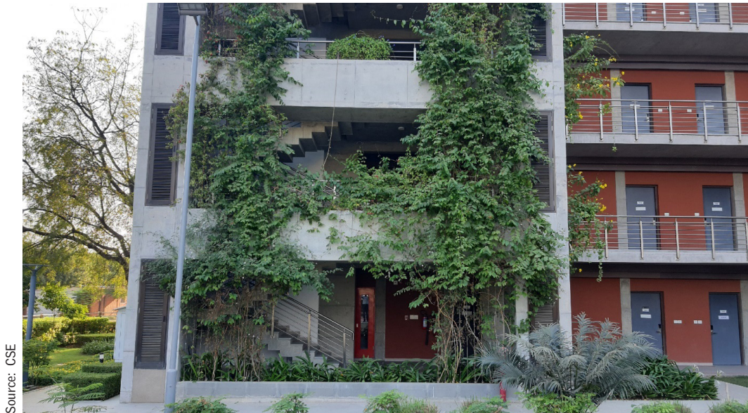
Vertical greening to block direct solar radiation and reduce ambient temperatures through evapotranspiration
