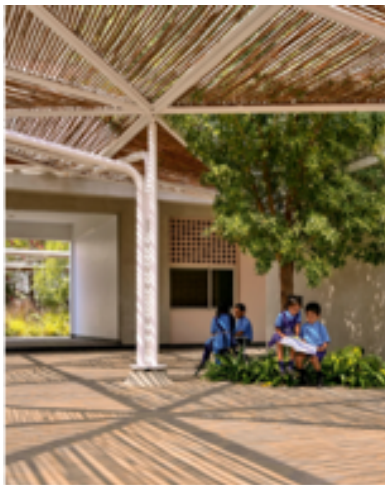
Sun shade constructed from bamboo for open spaces in Penna Foundation School, Talaricheruvu, Andhra Pradesh
