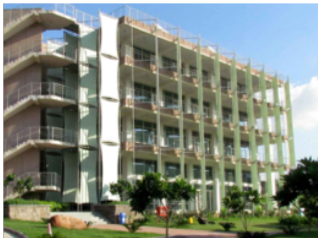
Vertical fins acting as sun shading device at IIIT Delhi
