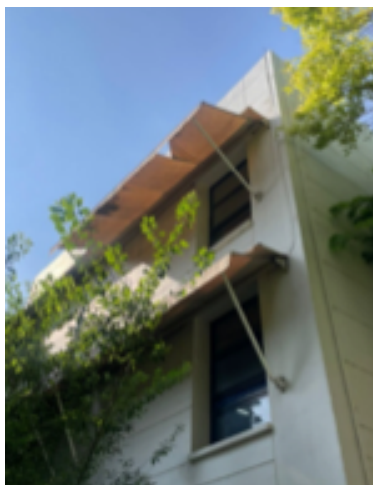
Retractable horizontal sun shading device over windows at CSE office, Tughlakabad, New Delhi
