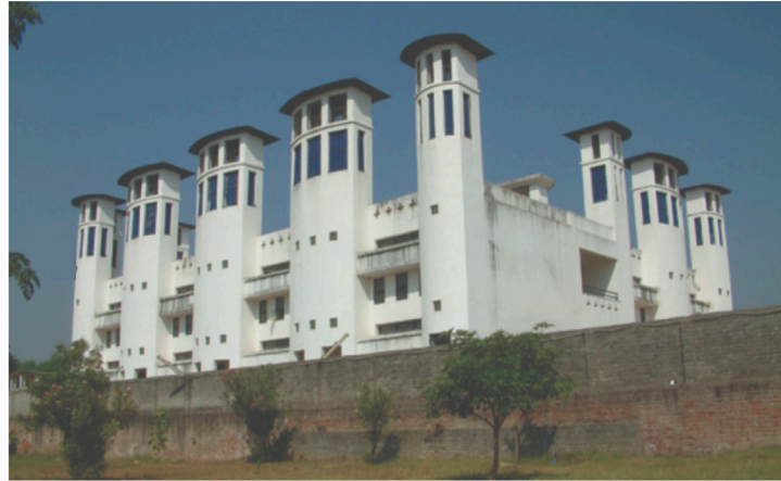
The section of direct evaporative cooling system (left); Air inlet and outlet shaft in Shri Swami Vivekanand Vidhya Vihar classrooms in Nadiad, Gujarat (right)
