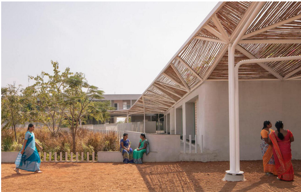
Bamboo shading devices retrofitted around the classrooms to reduce solar heat gain, in Penna Foundation School in Andhra Pradesh
