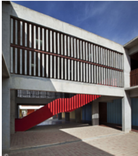
Terracotta Jaali (left) and vertical shading devices (right) adopted in Delhi Public School, Bengaluru to minimize direct solar heat gain
