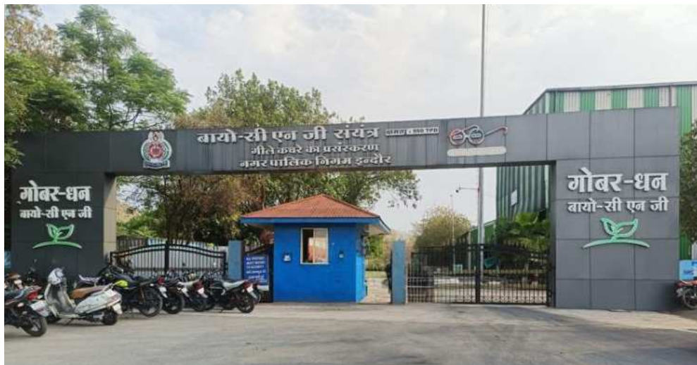
Bio-CNG Plant at Devguradia, Indore
