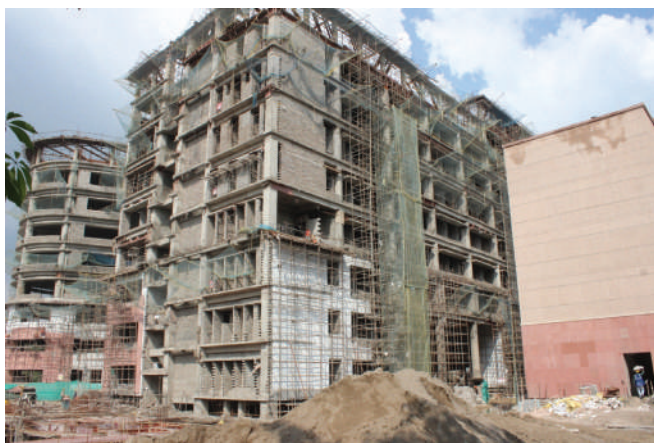
The Supreme Court Annexe building used 1.8 million recycled C&D waste blocks
