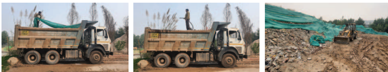
Covered transportation (left), wetting of debris (middle) and covered storage (right)
