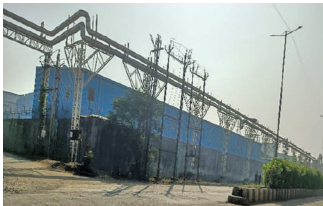
Common boiler pipeline laying
