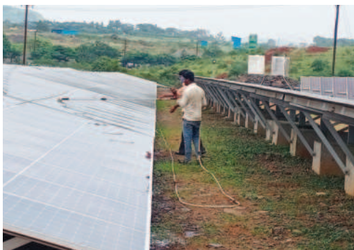
Cleaning solar panels
