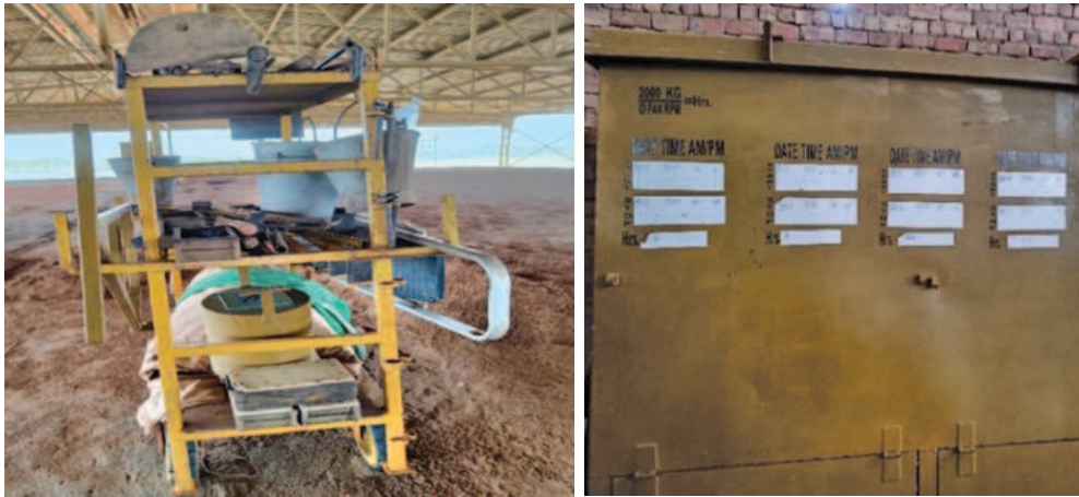
Fuel feeding process with temperature measuring instruments and record keeping
