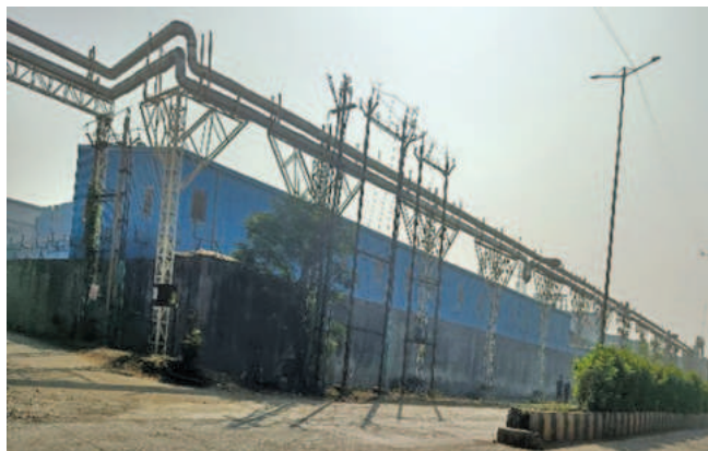
Common boiler pipeline laying
