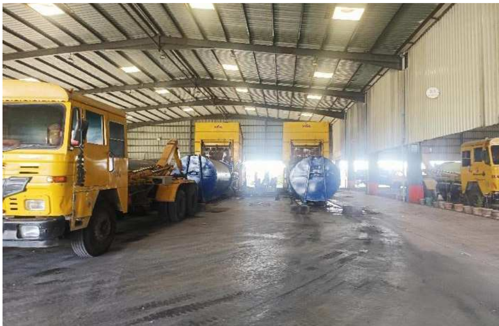
Waste processing in site
