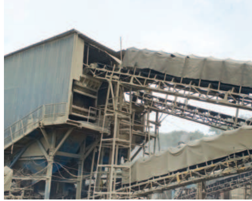
Covered secondary crushing units
