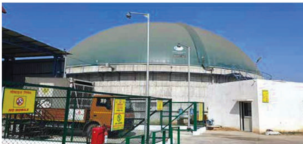
Biogas digester with a total capacity of four tonnes per day (TPD)
