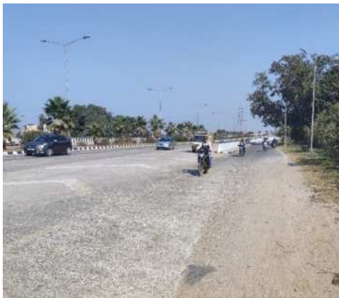
Ring road construction at Sarnath, Varanasi
