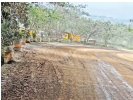
Regular sprinkling done on the road
