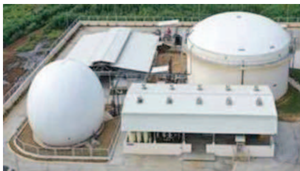
Overview of the Banaskantha CBG plant
