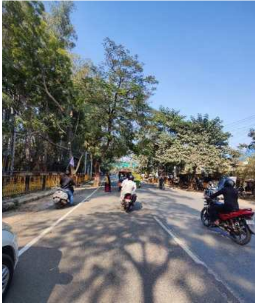
End-to-end road pavement at Hiranpur, Varanasi
