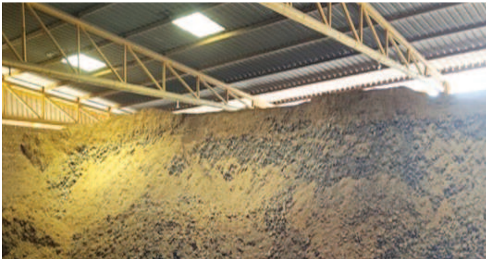
Fuel storage area with natural light access from the shed
