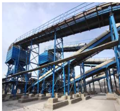
Covered conveyer belt
