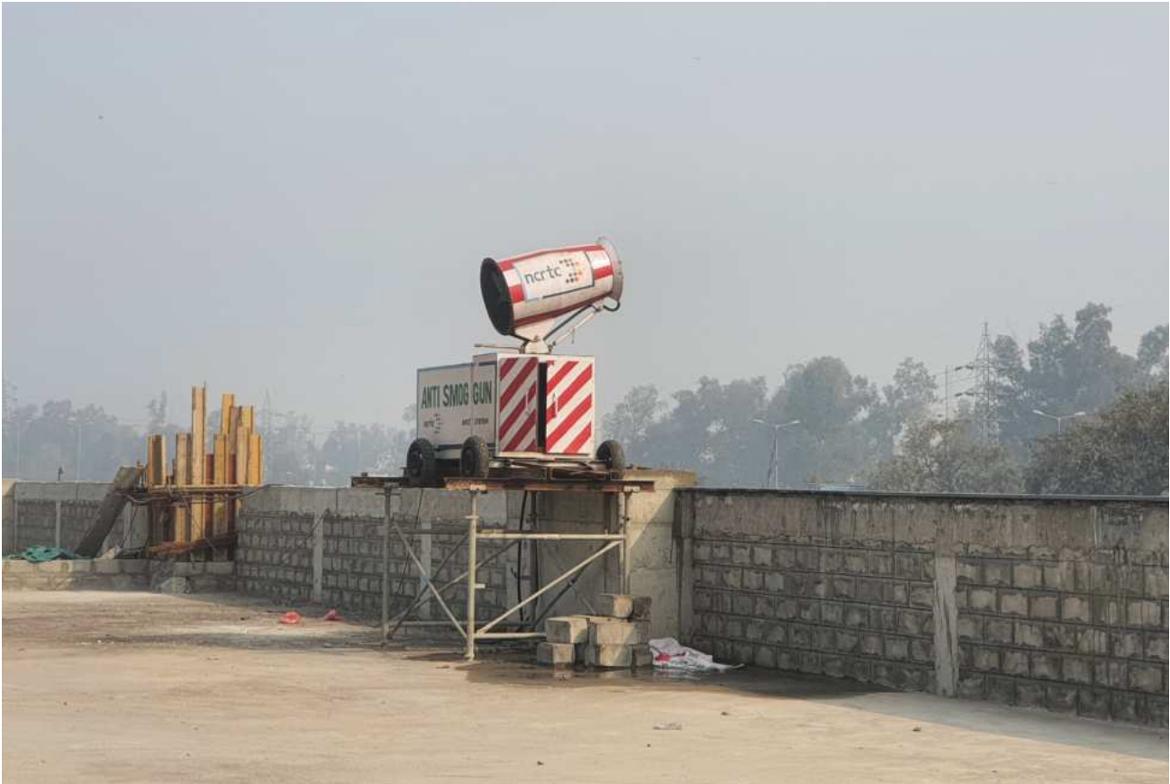
Anti-smog guns kept at high elevation of buildings
