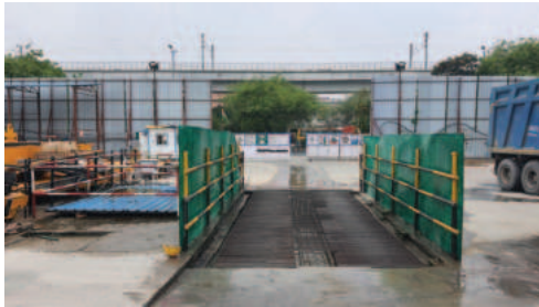
Wheel washing stations at a DMRC site entrance
