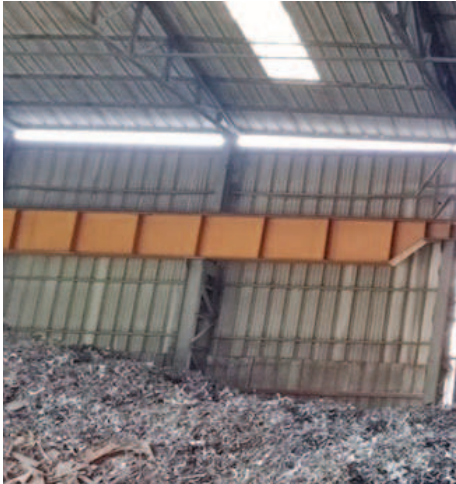
Raw material stored in covered space
