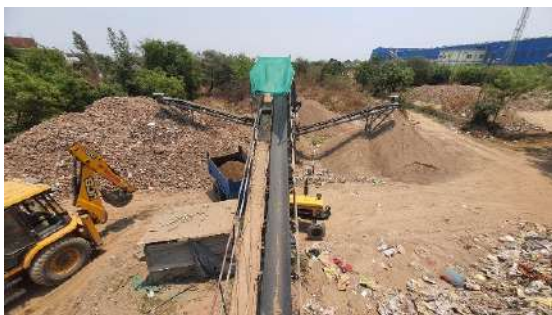
Recycling of C&D waste in Ramana
