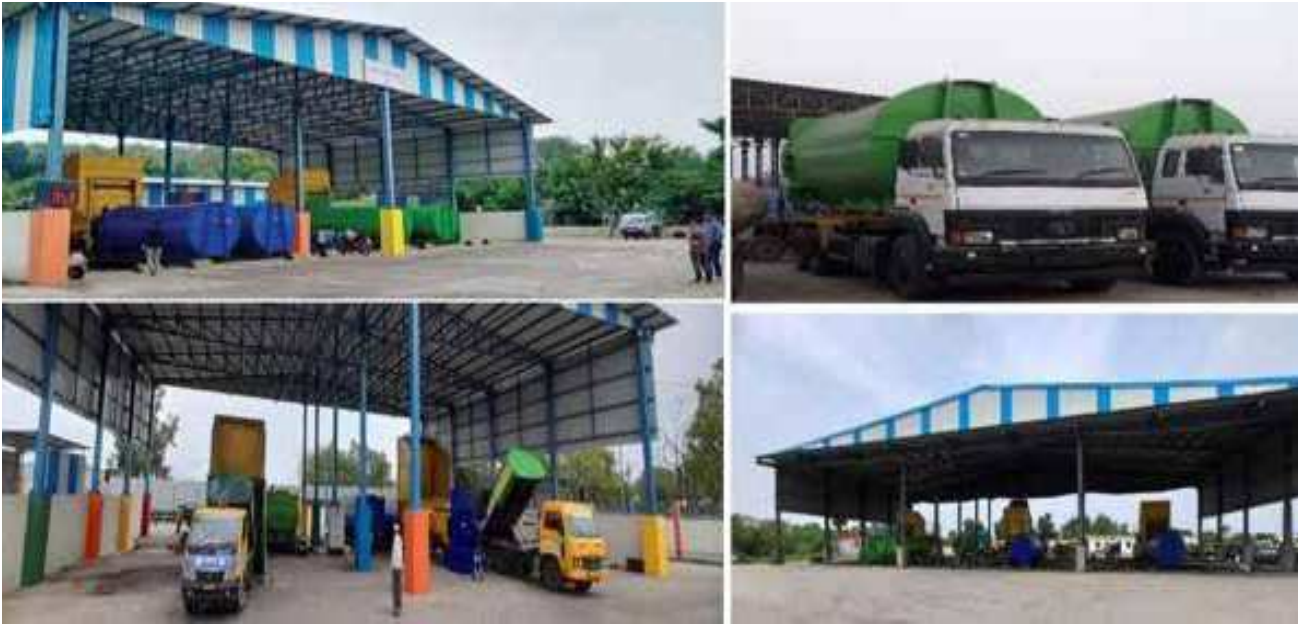
Waste transfer station in the city
