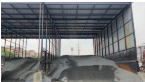
Material handling taking place within enclosure
