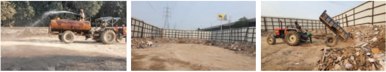
Wetting of roads, wind barrier, and low drop height at the collection centre
