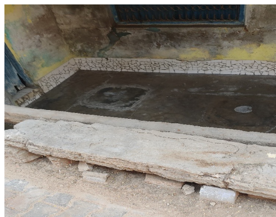
A containment at a lower ground level due to a recent levelling of roads
