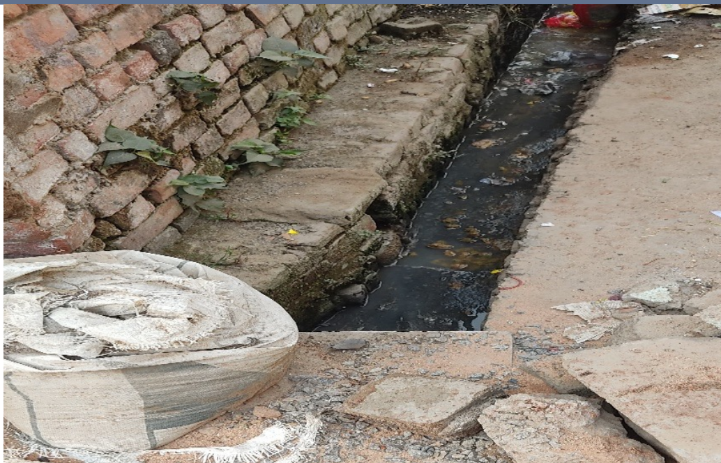
Households discharging domestic wastewater into an open drain
