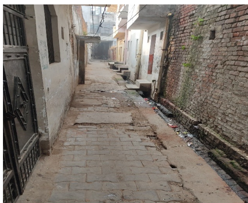
Areas with narrow lanes have prominent semi-lined systems and toilets discharging directly into open drains
