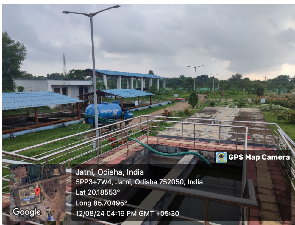
An overview of Jatni FSTP showing STT, ABR, SDBs and sludge storage shed
