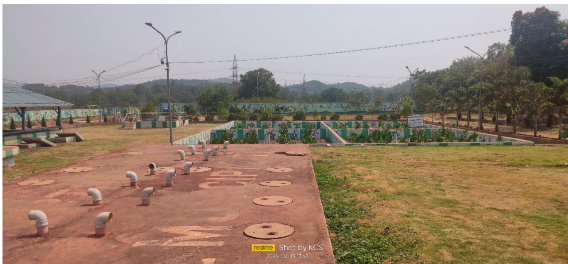
Anaerobic baffled reactors (ABR) and planted gravel filter beds at Barbil FSTP
