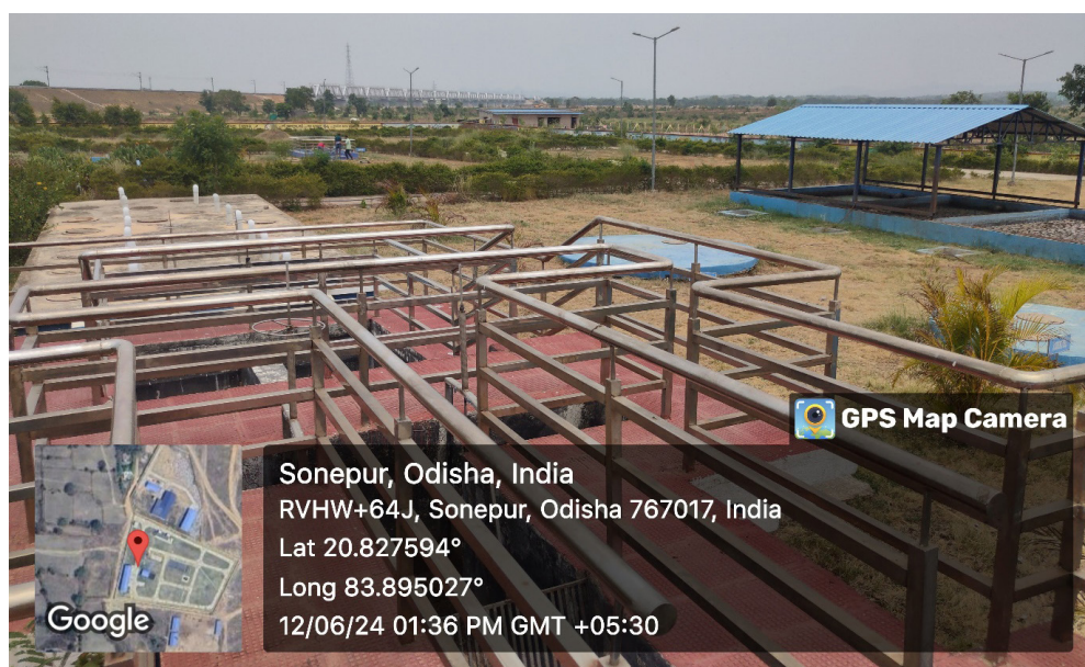
Settling thickening tank, anaerobic baffled reactors (ABR) and unplanted sludge drying beds at Sonepur FSTP
