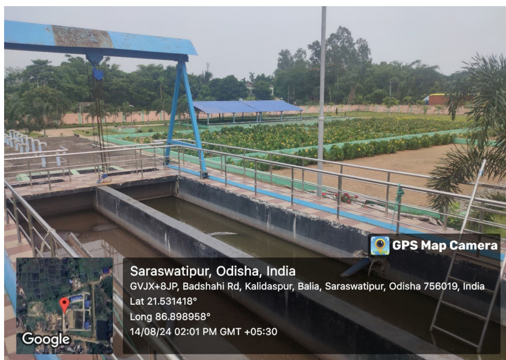
The STTs, ABR, PGF beds and SDBs at Balasore FSTP
