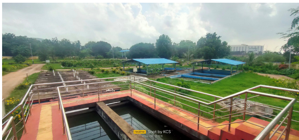
An overview of Khordha FSTP showing STT, ABR and SDBs
