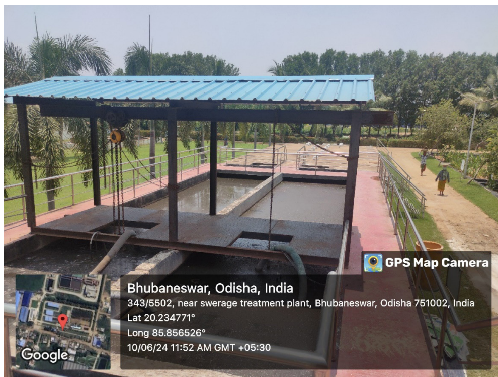
Settling thickening tank at Rokati FSTP, Bhubaneswar
