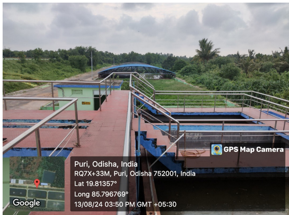
The STTs and SDBs at Puri STP co-treatment plant Source: CSE
