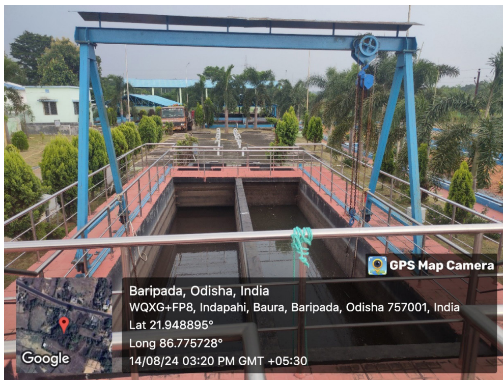
STTs and ABR at Baripada FSTP
