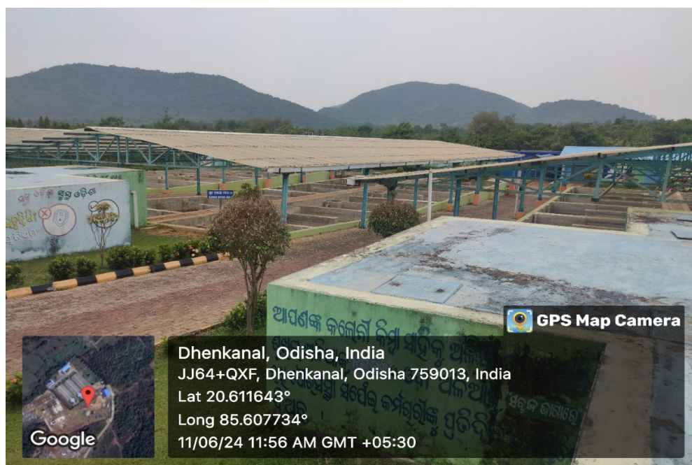
Anaerobic stabilization reactors and series of unplanted SDBs at Dhenkanal FSTP
