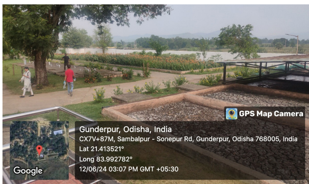
An overview of Sambalpur FSTP showing SDBs, ABR and PGF beds.
