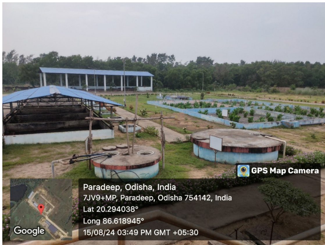
PGF beds, unplanted SDBs and sludge storage shed at Paradeep FSTP
