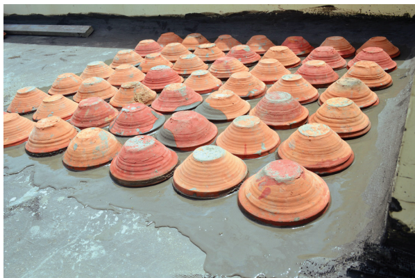
Inverted earthen pots being used for roof insulation in a demonstration project in Indore.
