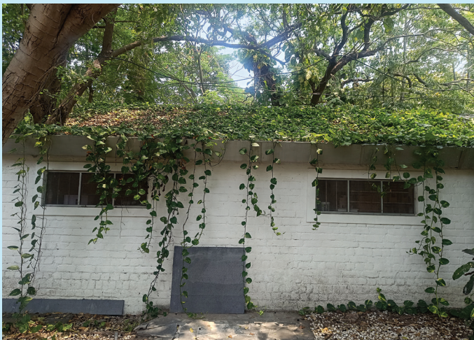
The Ovoid office with GI sheet roofing layered with green roof (left). Pockets woven into geo-fabric filled with soil (right) act as media for the vegetation, laid over the roof
