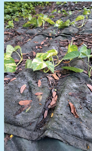
The Ovoid office with GI sheet roofing layered with green roof (left). Pockets woven into geo-fabric filled with soil (right) act as media for the vegetation, laid over the roof
