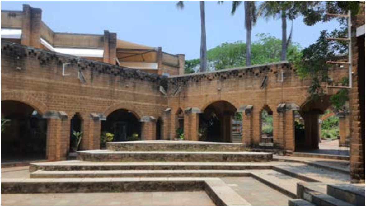
The visitors' centre in Auroville, Tamil Nadu, uses compressed earthen blocks
