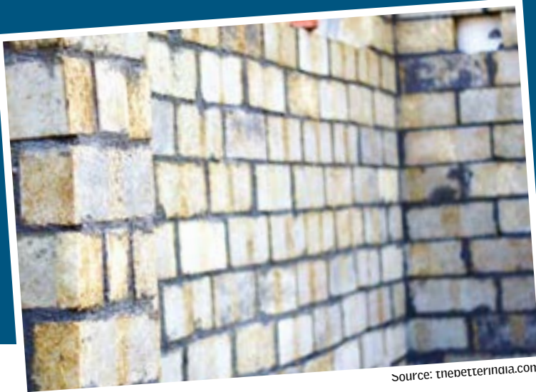
A guard cabin based on bio-bricks is constructed in IIT Hyderabad
