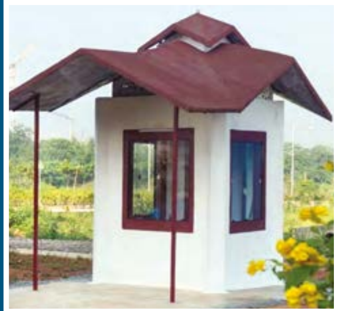
A guard cabin based on bio-bricks is constructed in IIT Hyderabad
