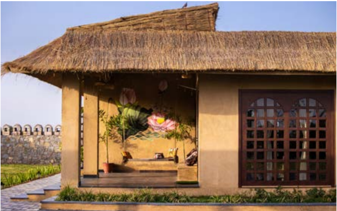
A house in Chittorgarh, Rajasthan, that uses thatched roof and rammed earth walls
