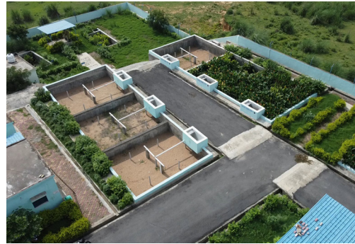
Chunar FSTP (10 KLD), commissioned in September 2022
