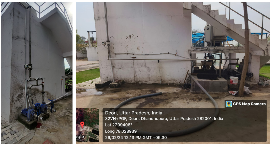
Before: Directly pumping the septage After: Pumps removed from the place, screen chamber constructed followed by pumping of septage
