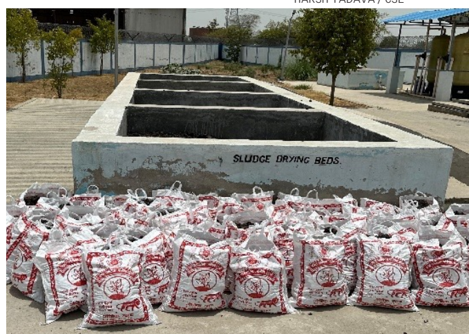
Pile-up of bags in which biosolids are stored in the absence of a storage room, Khurja
