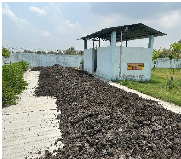
Biosolids stored on the pathways when the storeroom is full in Amroha city
