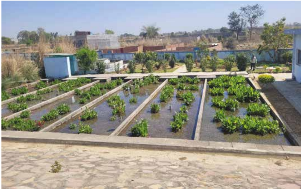
PGF initiates both physical and biological treatment of the effluent
