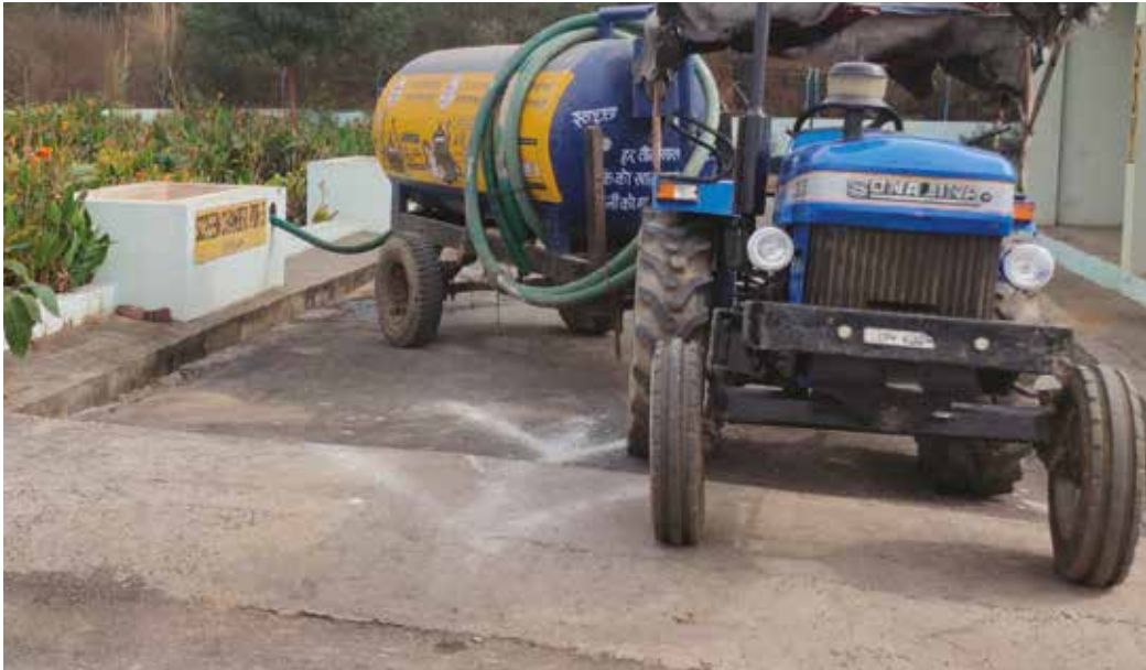
Desludging of FS in the screening chamber, further FS has been transferred to PDB initiating solid- liquid separation
