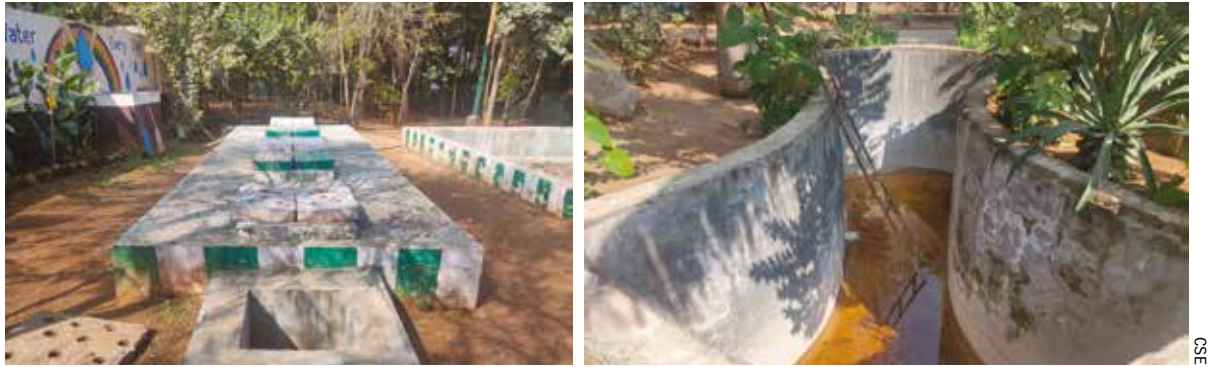
Secondary and tertiary treatment modules in Jhansi (6+12 KLD)
