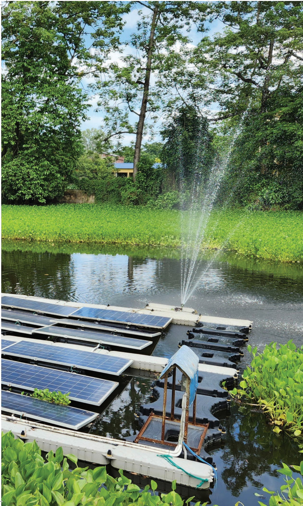
Floating solar panels mounted on a water surface, operating alongside an aeration system
