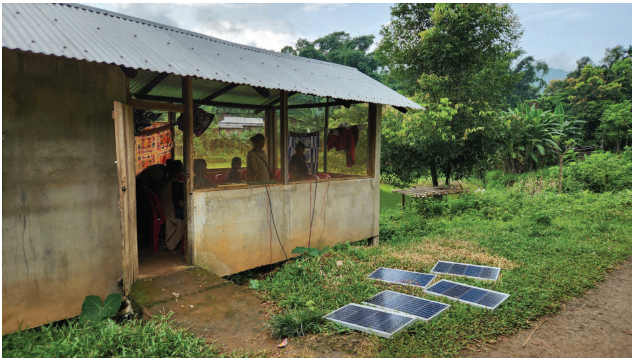
Community shed with portable solar panels kept outside to power the spinning machines
