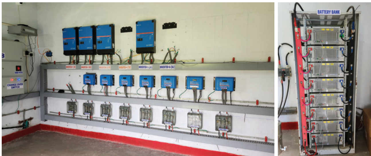
Inside the control room where inverters and lithium-ion batteries manage the village's load
