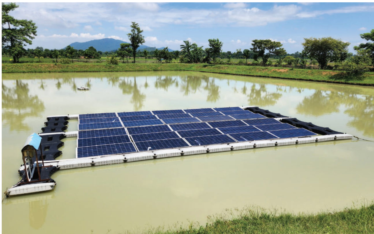
Floating solar panels installed on a pond of Kalong–Kapili Integrated Aquaculture Centre to power fish farming
