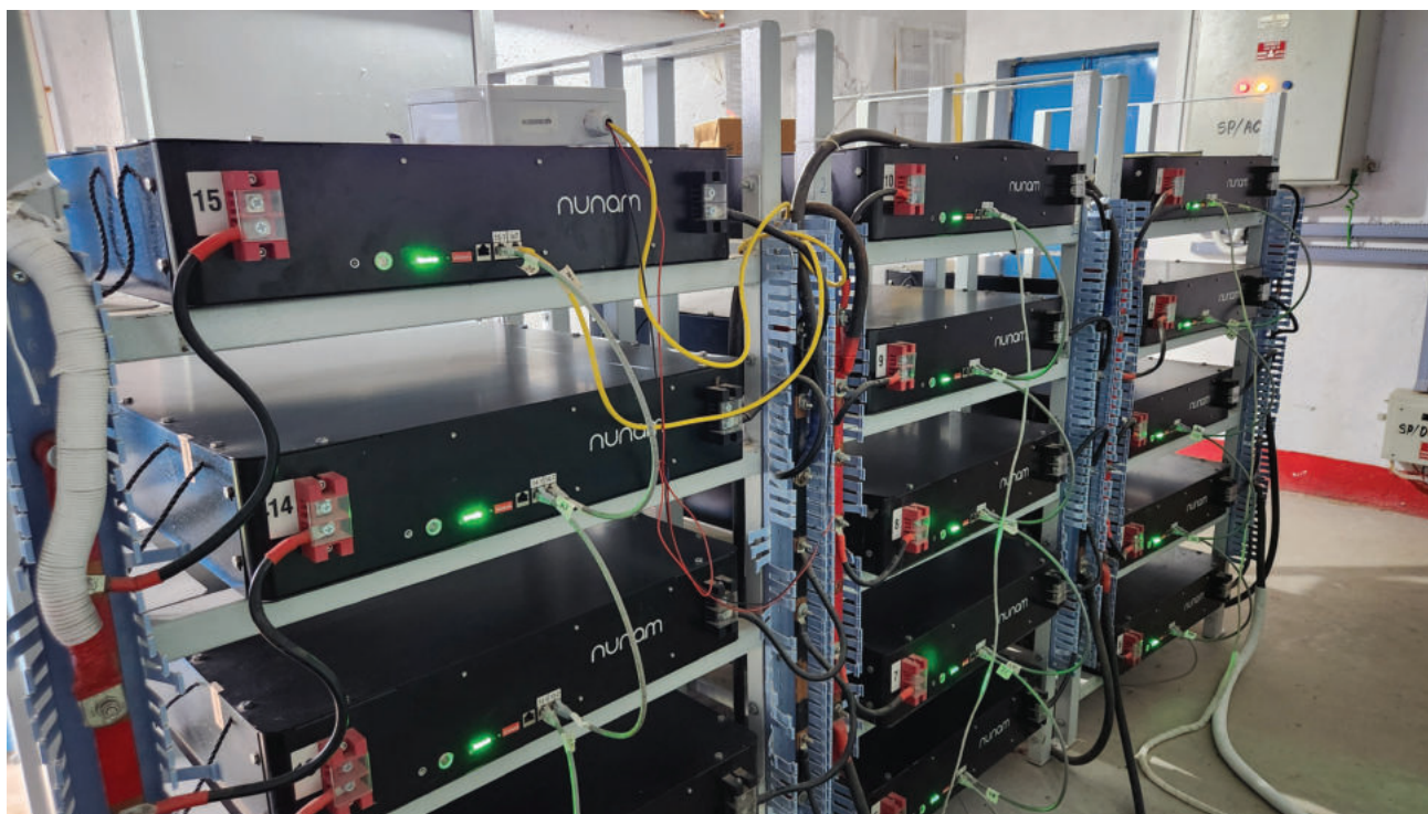
Rows of lithium-ion batteries storing energy to keep the mini-grid running through the night
