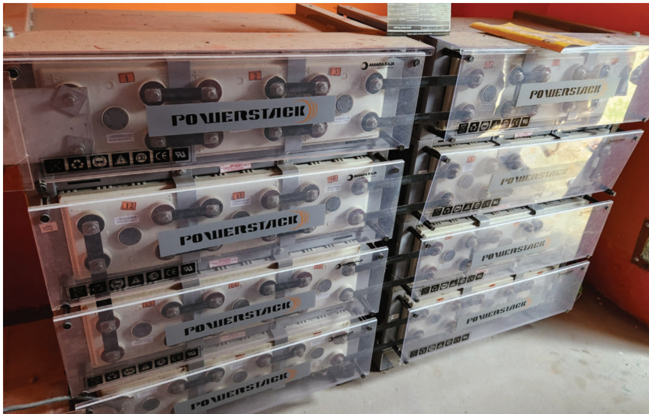
Stacked battery bank forming the backbone of mini-grid in Sugadongar
