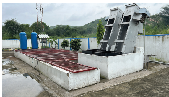
FS receiving unit with screens and effluent treatment modules at Kishangarh Bas FSTP;
