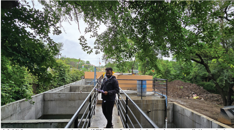
A 1-MLD sewage treatment plant (STP) near Pashan Lake to clean the pollution entering the lake
