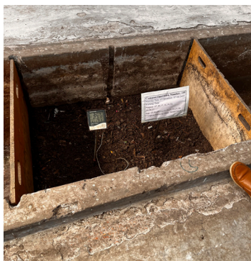
Sakhipur FSTP windrow pits for co-composting
