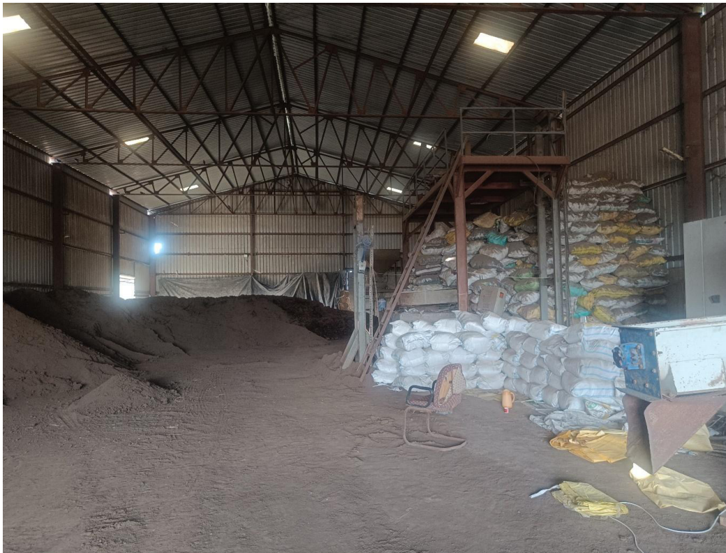
The plant's FOM storage and packing area
