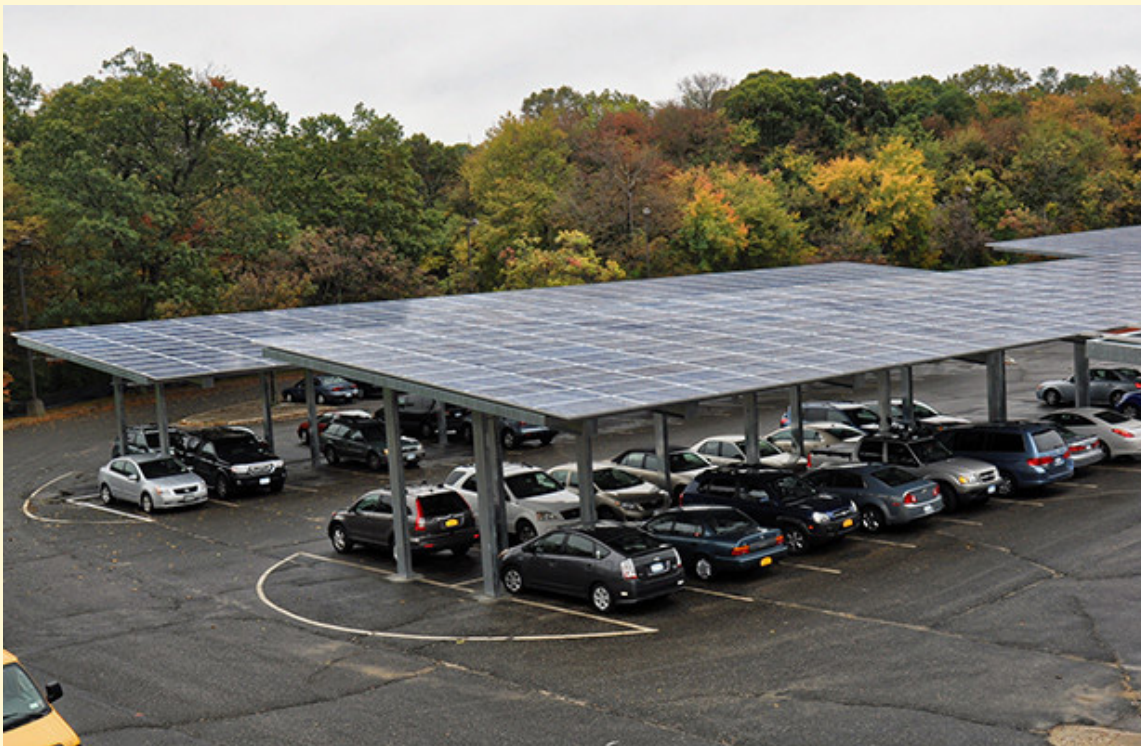
Retractable umbrella canopies in an educational institute in Australia (top), Solar panels used as shading devices over car parking (bottom).
