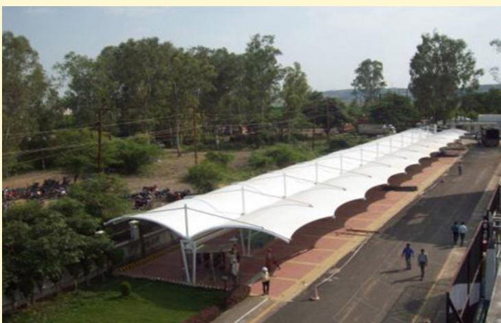
Different approaches for shading (left) Tensile fabric canopy roofed car park at Mysuru, Karnataka (right) Metal frame with wooden trellis allowing vegetation to grow over
