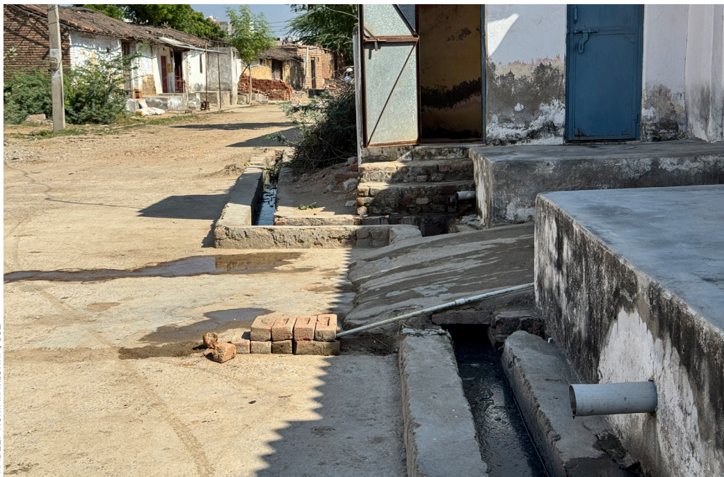
Greywater from kitchen and washing area inside the house flowing into the open drains, village Pratapgarh, block Rani, Pali district (Rajasthan)
