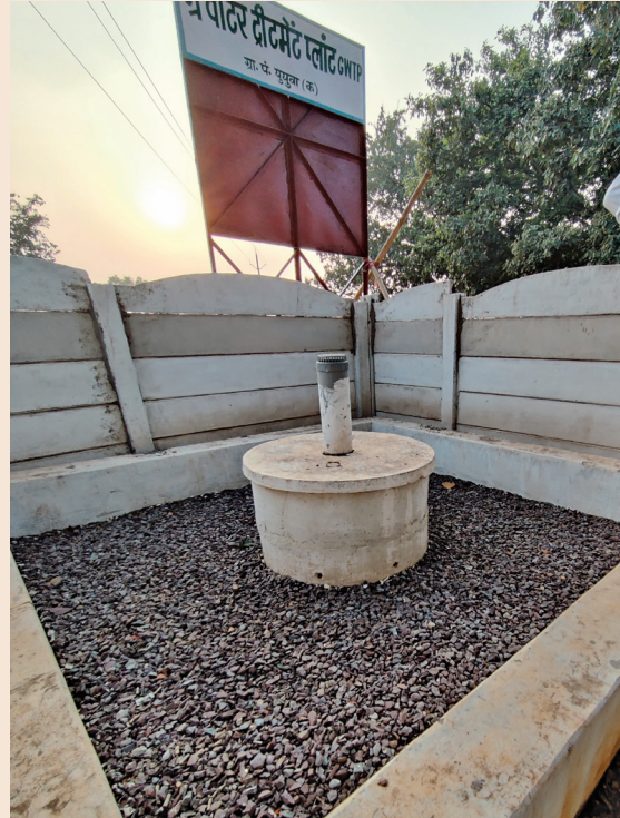
Soak pit in Ghughwa greywater treatment plant
