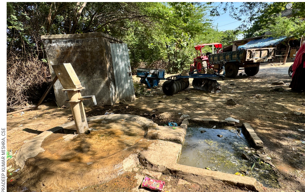
Soak pit in disuse and without silt chamber in Berdi village, Bali block
