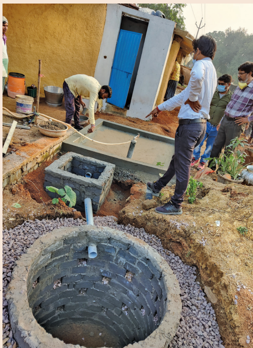
Household-level modified soak pit with a platform and silt chamber in Durg district
