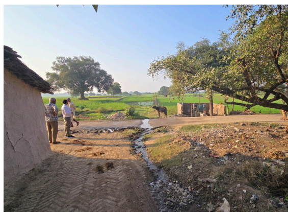
A drain in Bhatia village, a small village in Jaspura block, ends up in agricultural fields. The image shows a disconnect in the segments of drains: while one part of the village has a drain, its lower elevation lacks one, leading to waterlogged roads. Communities report that these drains are made in small parts by the gram panchayat.
