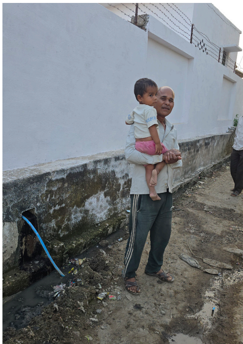
Drinking water pipeline passing through a greywater drain in Mohan Purwa village, Badokhar Khurd block. In case of leakage, the greywater would contaminate the drinking water supply (left). Drain or no drain? Sadha village, Naraini block (right).
