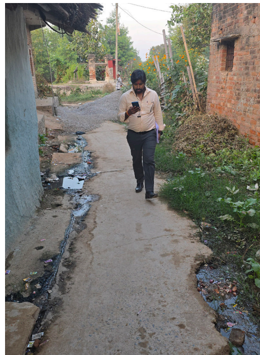
Drinking water pipeline passing through a greywater drain in Mohan Purwa village, Badokhar Khurd block. In case of leakage, the greywater would contaminate the drinking water supply (left). Drain or no drain? Sadha village, Naraini block (right).
