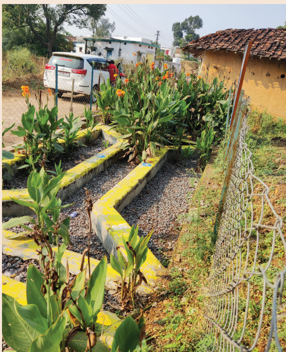
Canna indica growing in the constructed wetland used to treat grey water at the community level in Patora
