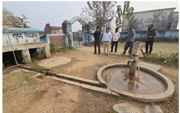
A proper functioning soak pit in a school in Samagra village, Baberu block
