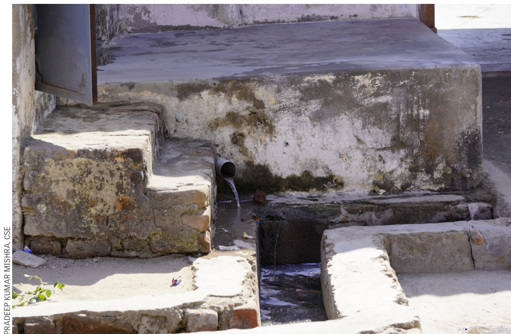
Greywater from households flows into open drains in Pratapgarh village, Rani block
