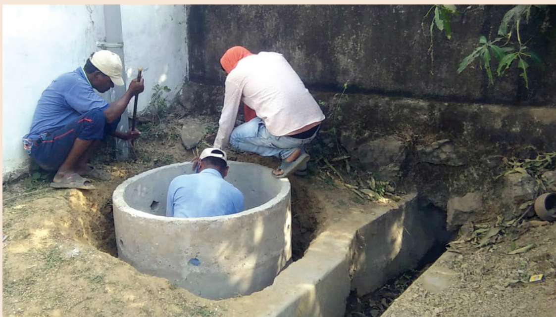
Construction of community-level leach pit in Patora village
