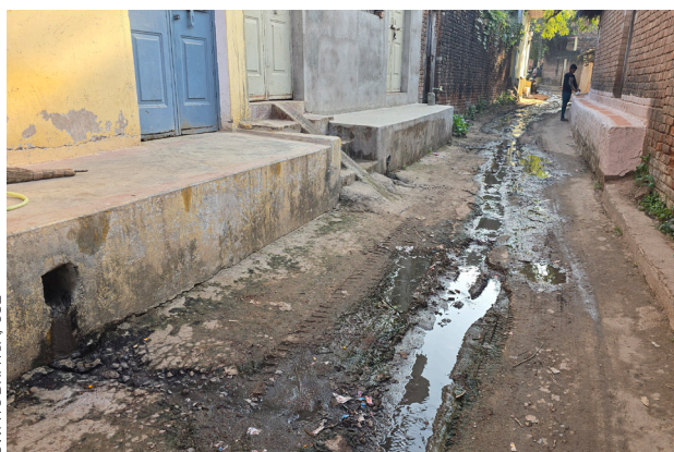
A drain in Bhatia village, a small village in Jaspura block, ends up in agricultural fields. The image shows a disconnect in the segments of drains: while one part of the village has a drain, its lower elevation lacks one, leading to waterlogged roads. Communities report that these drains are made in small parts by the gram panchayat.
