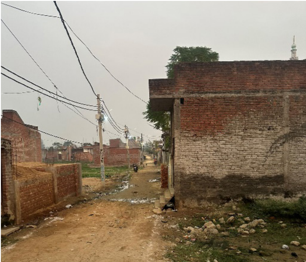
Ward 32 with areas having no wastewater drains
