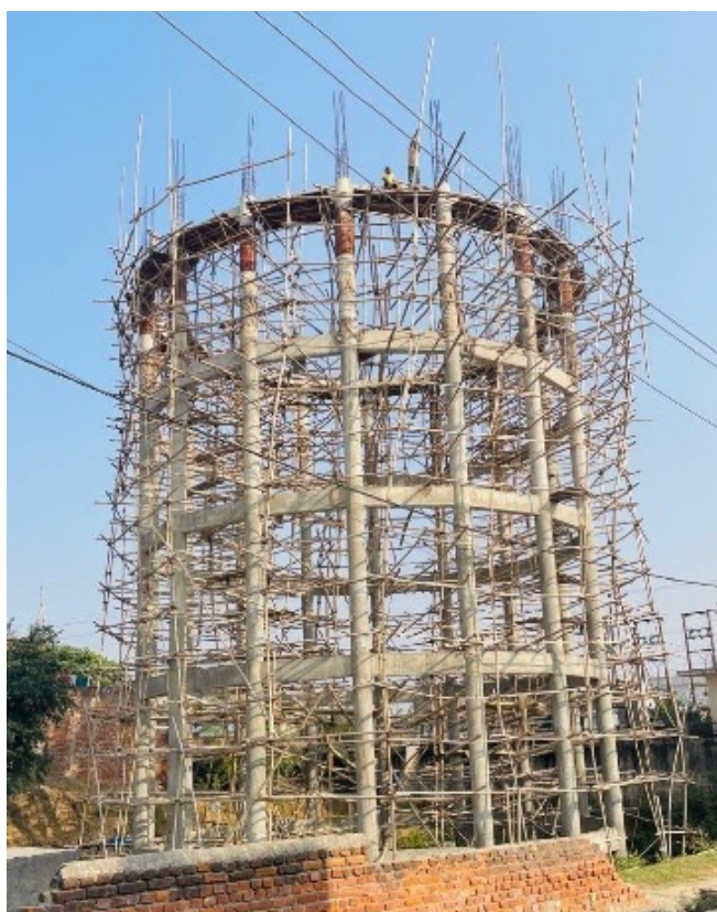
Under construction overhead tank in Ward 6
