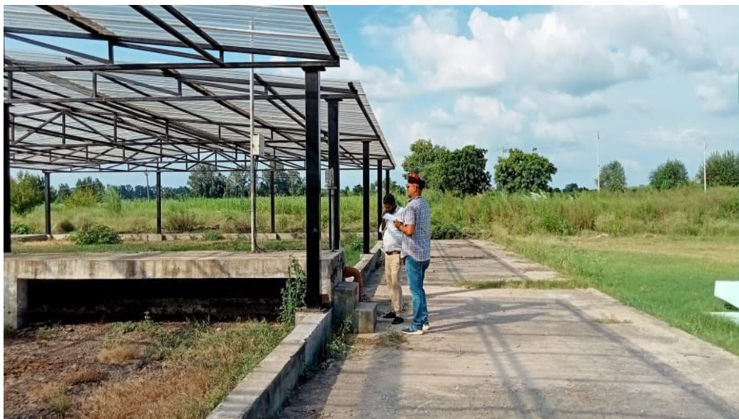
20 KLD co-treatment plant, Bijnor
