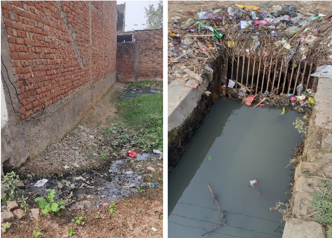
Wastewater accumulation in empty plot (left) and wastewater interception point in Ward 7 (right)
