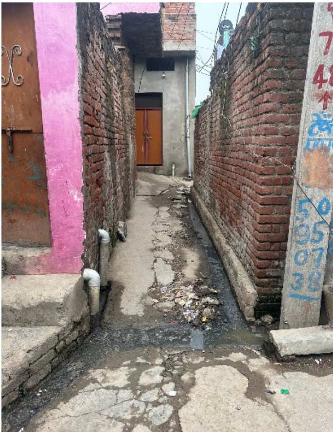
Narrow lanes where mechanical desludging is not possible in Ward 13
