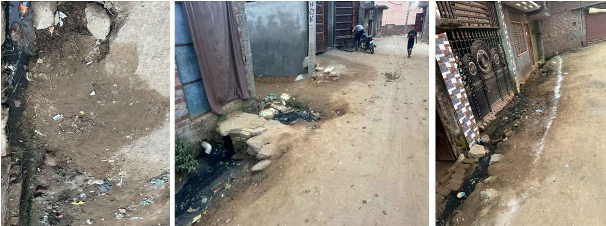
Household wastewater going on open ground (left); kachha drains outside households (middle); no roads and drains (right)
