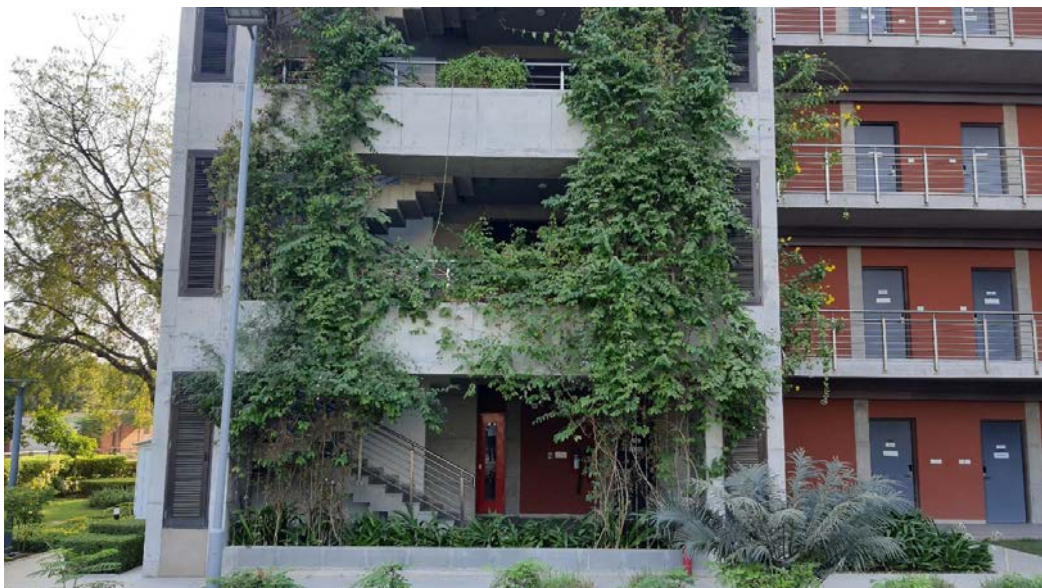
Vertical greening to block direct solar radiation and reduce ambient temperatures through evapotranspiration.
