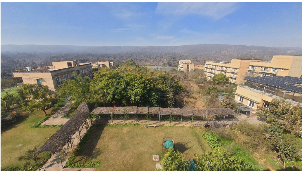
Tensile fabric canopy (top); metal frame with wooden trellis vegetation (bottom)
