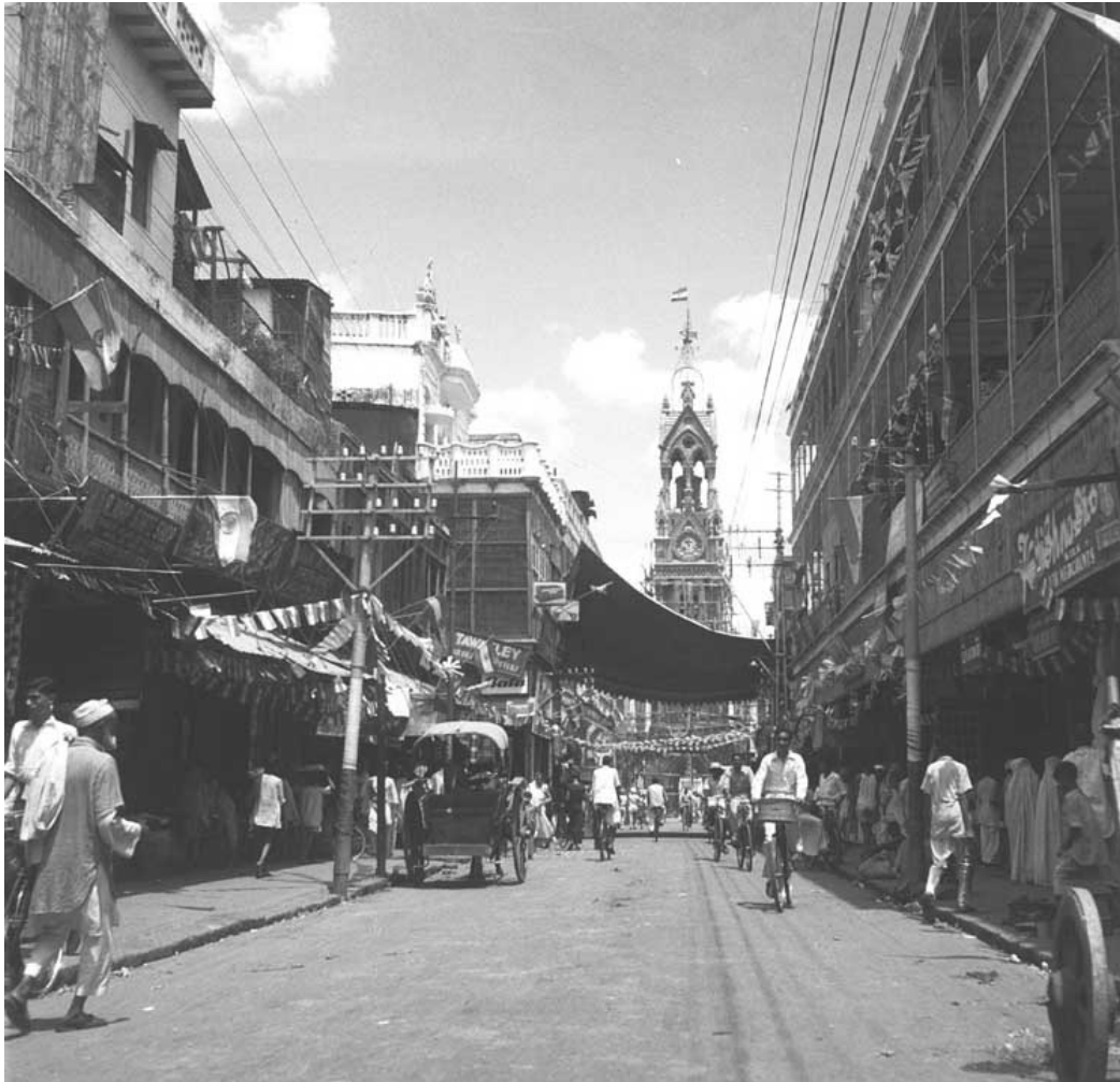
Chandni Chowk, Delhi, in 1947. A combination of shaded pathways, canopies and fabric-enhanced outdoor thermal comfort.
