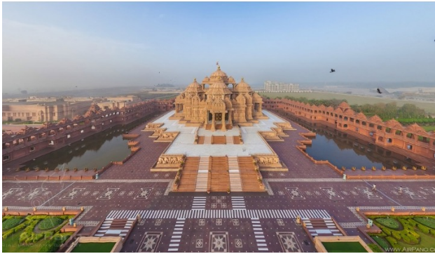
High reflectance stones used for paving in Akshardham temple, Delhi (left); high reflectance paint used over concrete Tirupati Balaji Temple, Delhi (centre and right) for cooler circumambulatory paths
