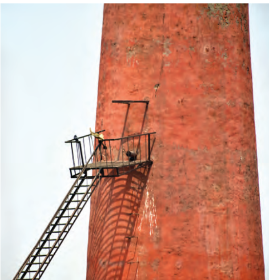
Damaged port hole and access ladder requiring maintenance
