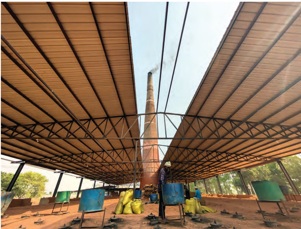
Brick kiln with proper shed providing better working environment for workers
