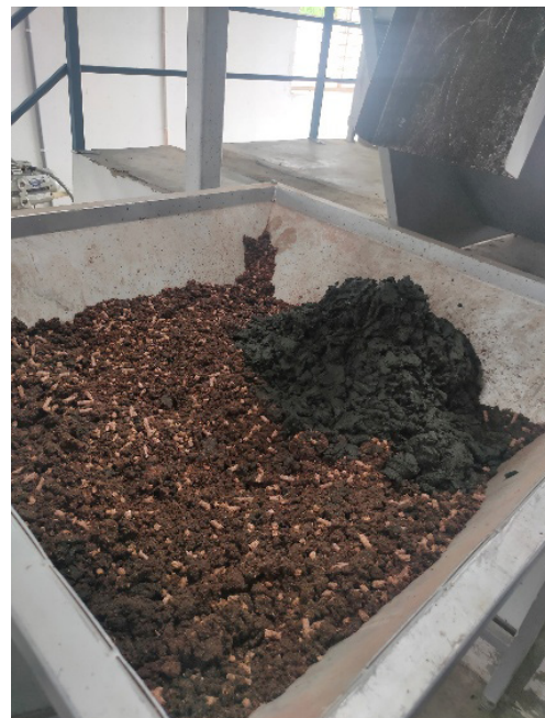
Dewatered biosolids mixed with wood chips at Kishangarh Bas FSTP
