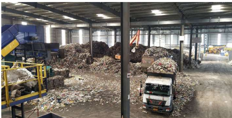
Material recovery facility in Indore
