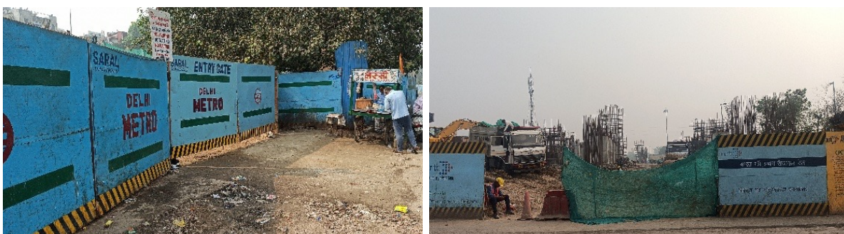
Entry-exit points for construction vehicles for metro construction
