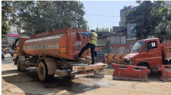
Water sprinkling on roads in and around the construction zone
