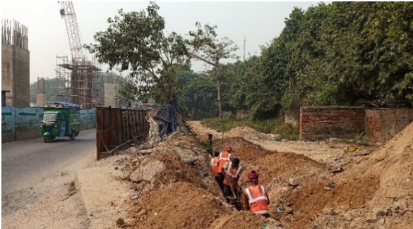
Excavation on the construction site
