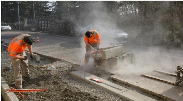
Dust during cutting and tiles laying
