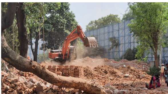
Material handling and uncovered material storage as a source of dust
