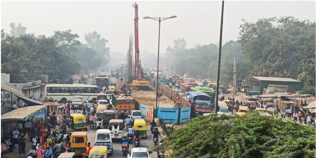
Congestion due to metro construction
