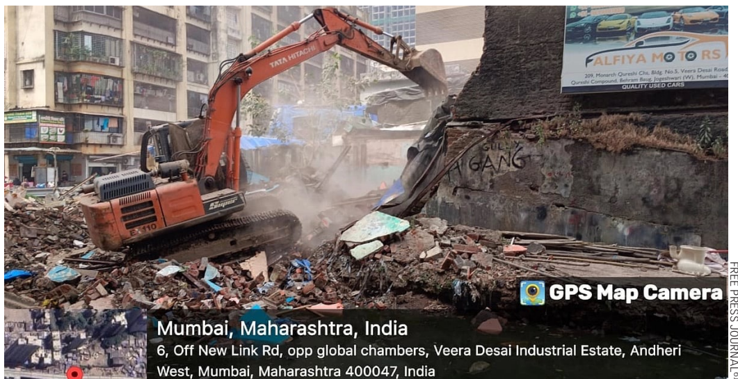
Demolition for metro construction in Mumbai
