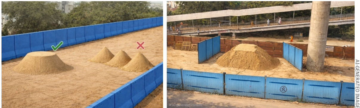
(a) Reducing surface area of stockpiles, and (b) Enclosing it with windbreakers reduces dust
