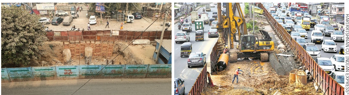
Tall wind barriers require space for foundations, but linear projects are often space-constrained
