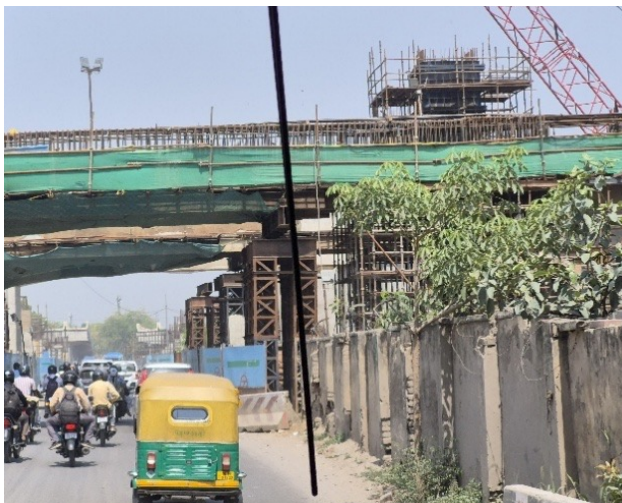
Dust barrier sheets used in metro construction
