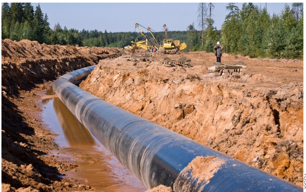
Laying of pipelines
