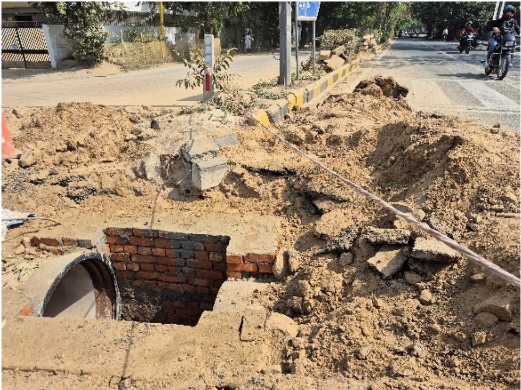
Excavation for stormwater drainage at a road junction
