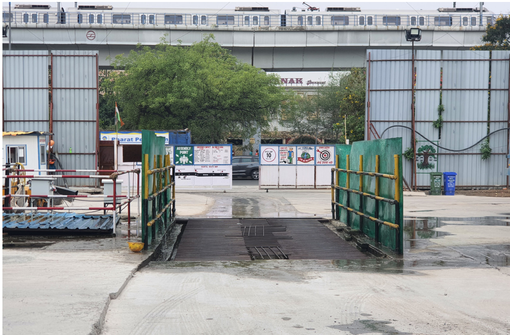
Wheel washing facility at Delhi metro site
