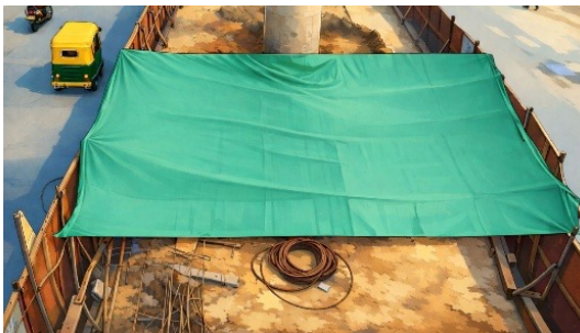
Cover sections of non-active construction sites
