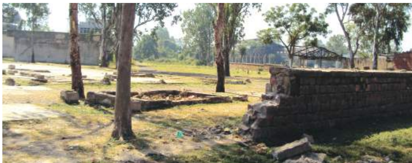
Broken boundary wall at UCIL, 2009
