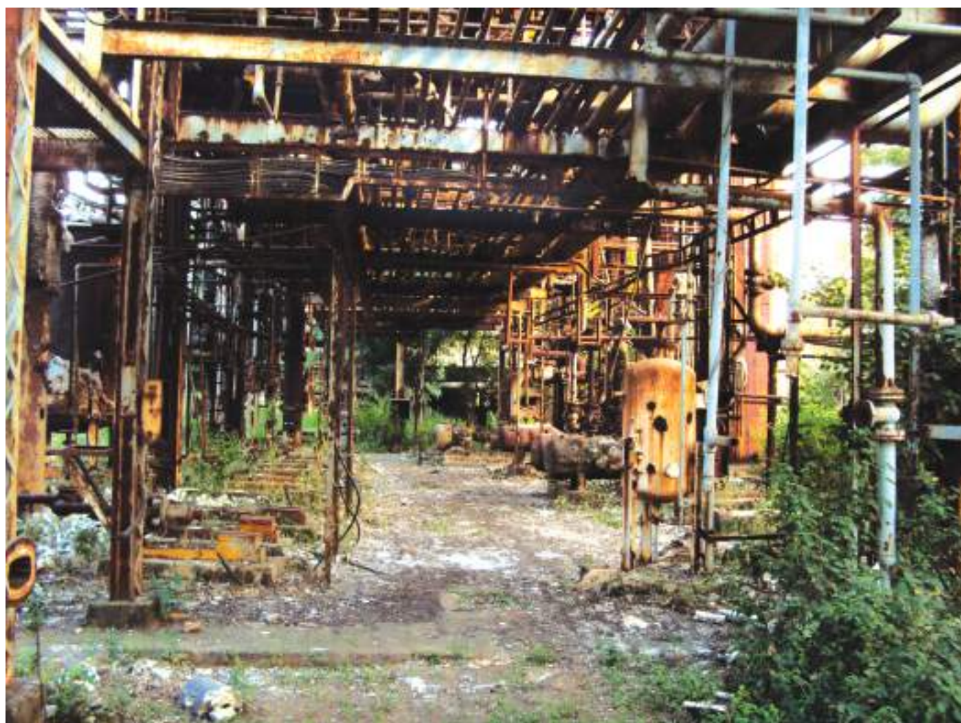
Plant machinery at UCIL, 2009
