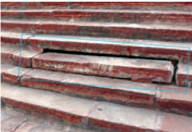
Entrance for manual O&M of first sedimentation Tank – stair step cover
