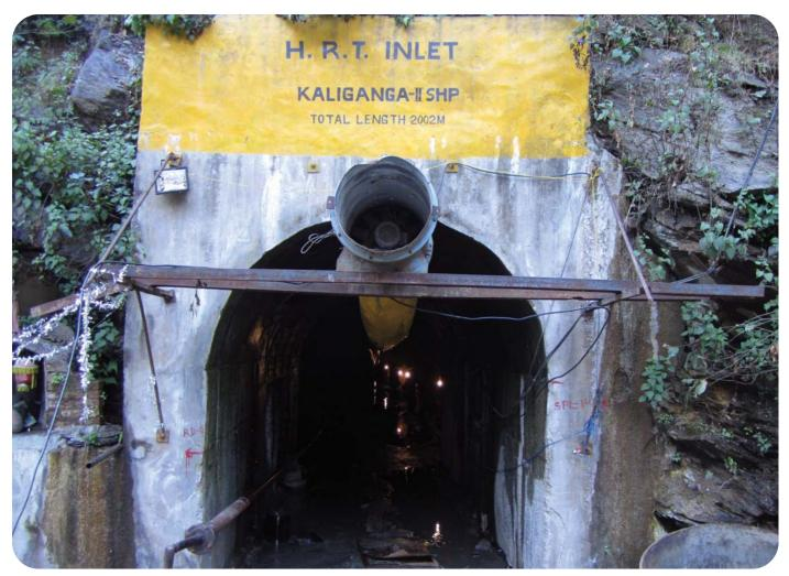
A 2-km long tunnel under construction, diverting the water for creating the necessary head at Kaliganga-II SHP plant
