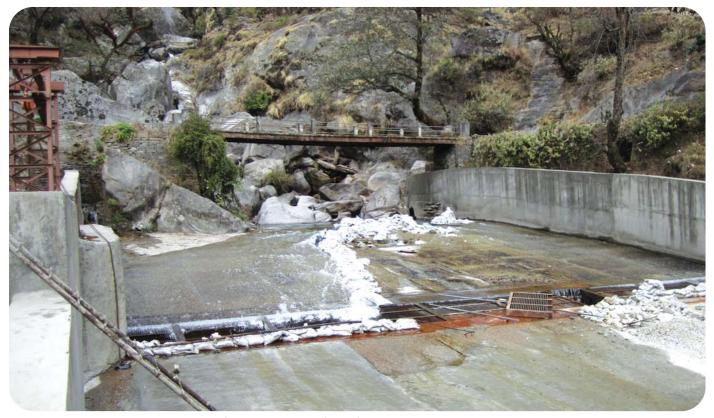
A trench-type diversion weir, with no provision for leaving a passage for the fish in a SHP project
