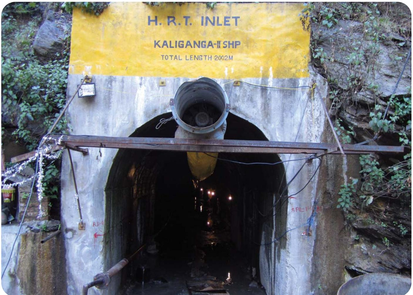
A 2-km long tunnel under construction, diverting the water for creating the necessary head at Kaliganga-II SHP plant
