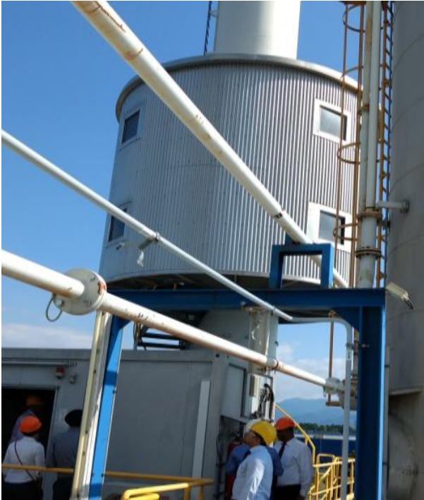
Well designed pollution-monitoring house/platform installed with stack (left); CEMS analyser house below the monitoring house at TREA, Breisgau
