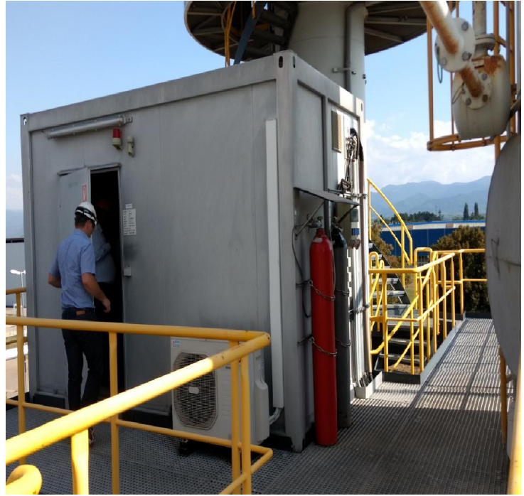
Well designed pollution-monitoring house/platform installed with stack (left); CEMS analyser house below the monitoring house at TREA, Breisgau
