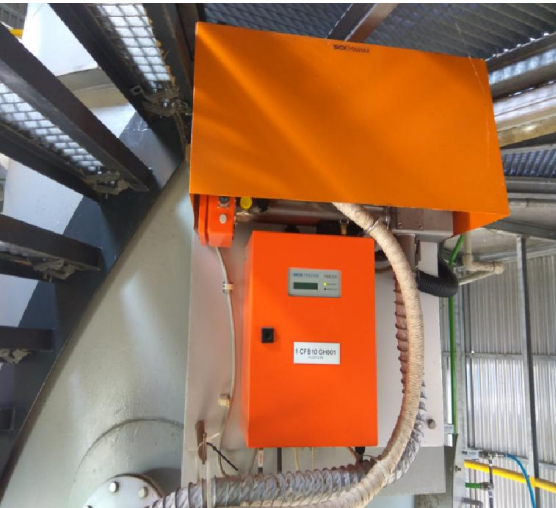
CEMS analyser installed inside the monitoring house/platform (L) and the team checking CEMS installation inside the monitoring house at TREA, Breisgau
