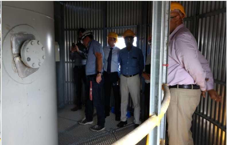
CEMS analyser installed inside the monitoring house/platform (L) and the team checking CEMS installation inside the monitoring house at TREA, Breisgau
