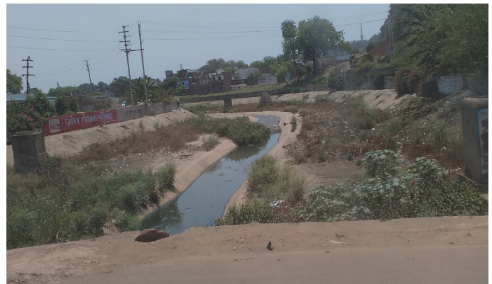
Figure 2: Outfall sewer along Swarnarekha River (Source: Shantanu/CSE, 2015)
