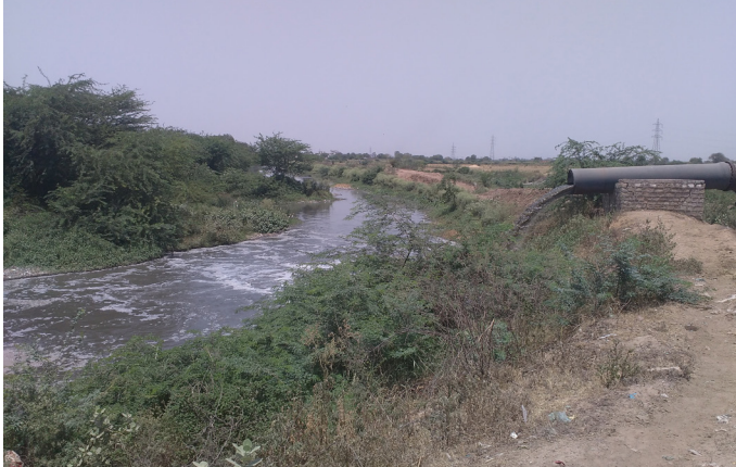
Figure 3: Indiscriminate discharge of wastewater into irrigation channel without treatment (Source: Shantanu/CSE, 2015)
