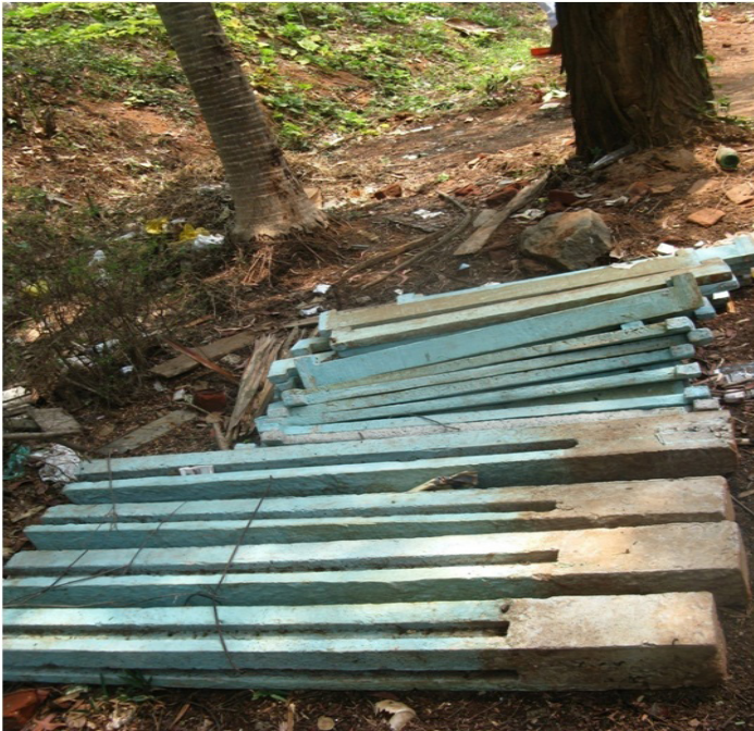
Figure 4: View of ferro-cement corner pillars and side bars dismantled
