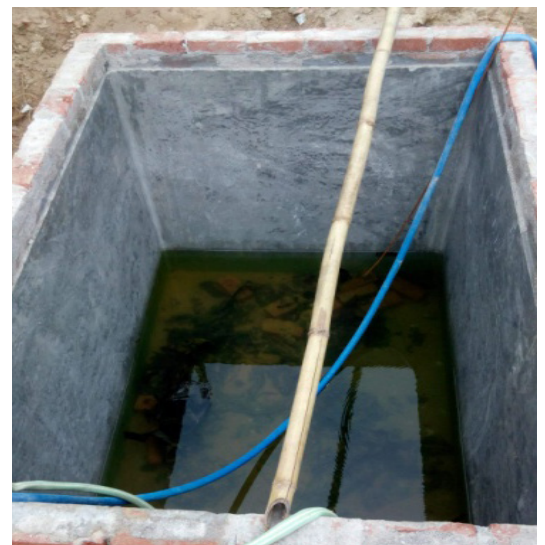
Figure 1: Septic tank of a household under construction
