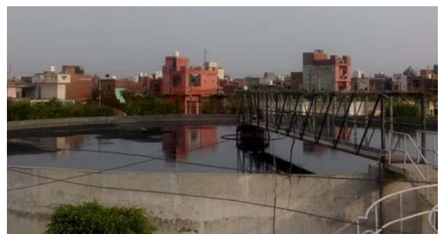
Figure 5: Sewage treatment plant working on MBBR technology
