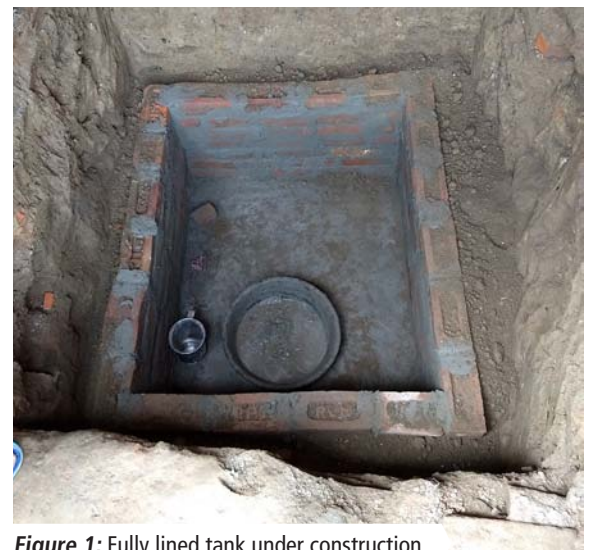
Figure 1: Fully lined tank under construction
