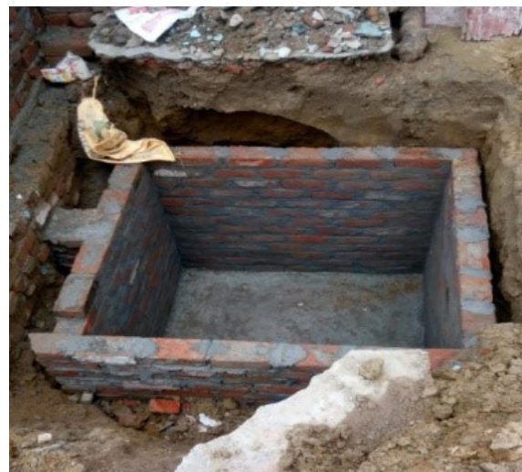
Figure 1: Fully lined tank under construction of a household
