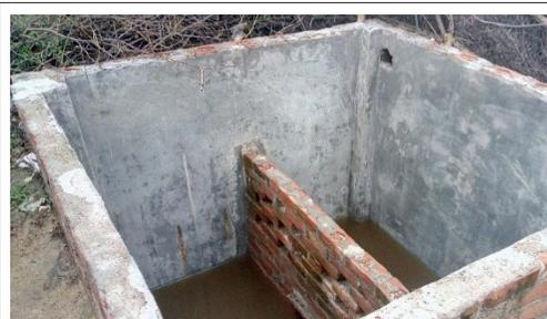
**Figure 5: Under construction septic tank in Lucknow**
