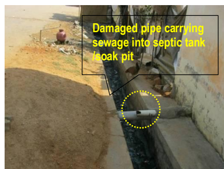
Picture 4: Drinking water pipe connected close to sewer drain at Nehru Nagar, Ward No. 56
