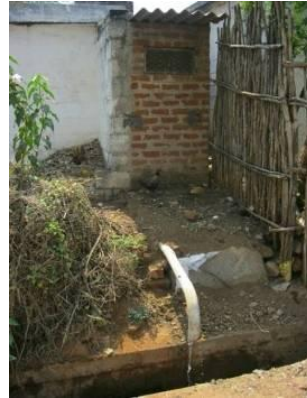
Sewer line directly let into open drain at Nehru Nagara, Ward No. 56
