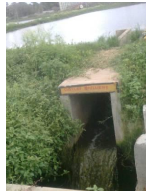
Picture 17: Outflow Point
