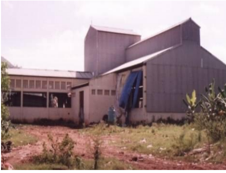
Picture 21: Waste management plant at Vidyaranyapuram
