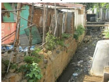
Picture 3: Household sewer lines connected to open nala at Gousiyanagar, Ward No. 59
