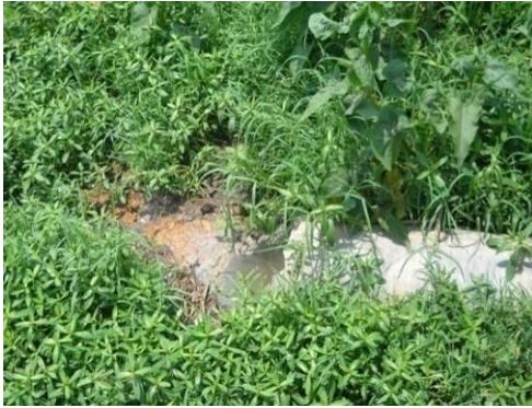
Picture 20: Sewerage outlet let into Kyatamarahalli lake
