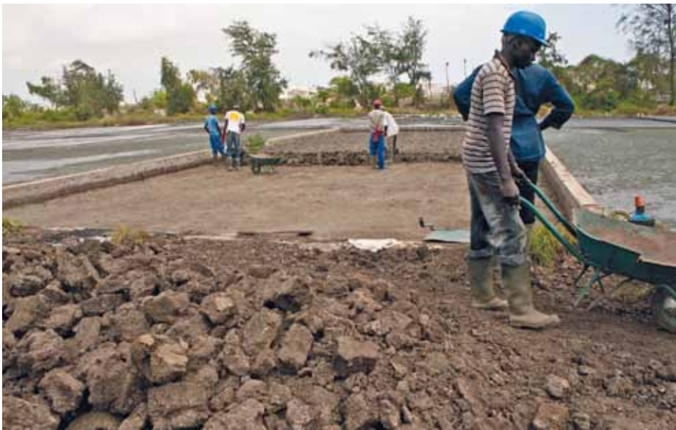
Figure 7.5 Removing sludge from unplanted drying beds at Cambérène treatment plant, Dakar, Senegal (photo: Linda Strande).
