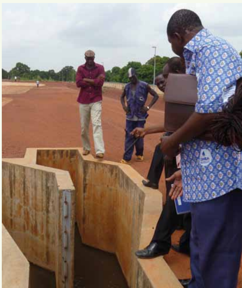
Figure 16.8 Inspection of an inlet, Burkina Faso (photo: Magalie Bassan).
