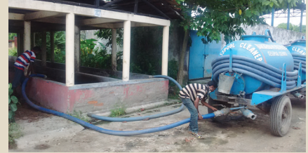
Septage management pictures depicting composting process at Bansberia
