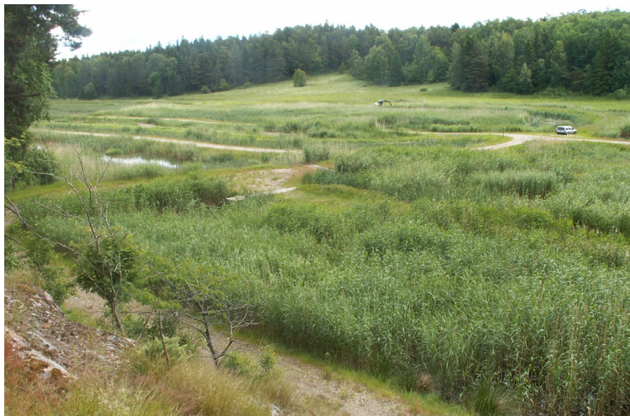
Figure 7.3 Wetland Alhagen with the first inlet wetlands and the alternately loaded West wetland (left), East wetland (background) and Inlet wetland (left of car) with bypass channel for stormwater between the pathways. Photo courtesy of Christer Svedin.
