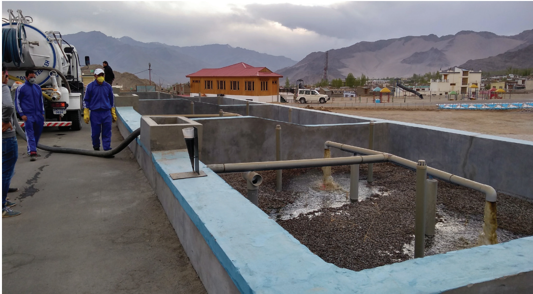
The fecal sludge treatment plant uses planted drying beds, into which the fecal sludge is discharged through a screen that captures any large inorganic solids (photo by CDD Society).
