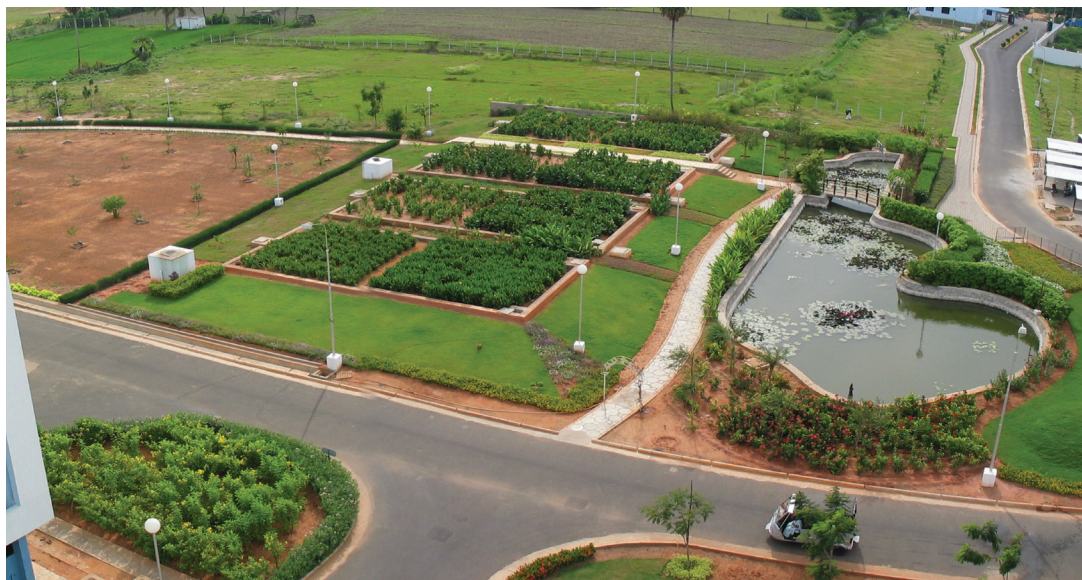
Planted gravel filter and polishing pond at Aravind Eye Hospital after construction (photo by Consortium for DEWATS Dissemination [CDD] Society).
