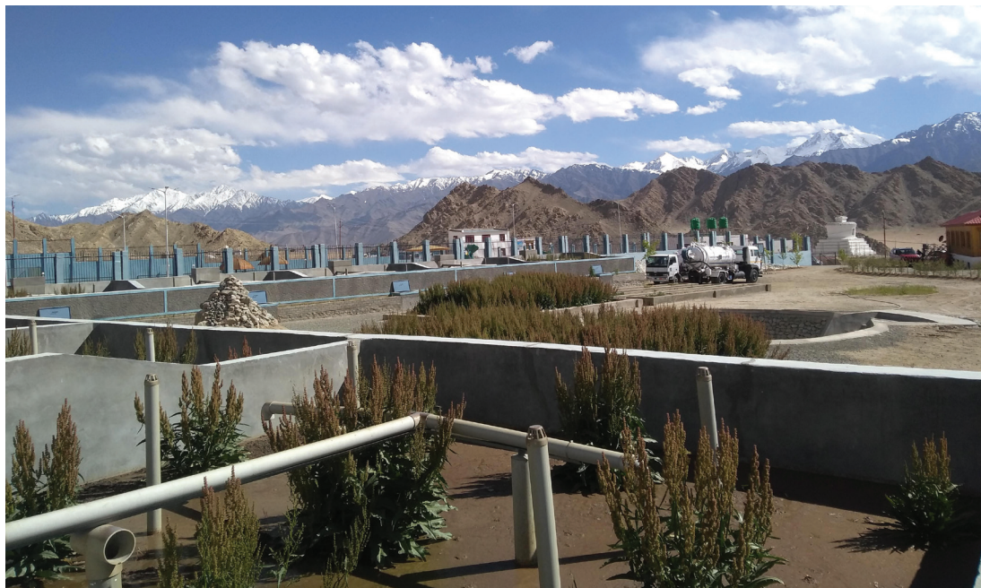
The fecal sludge treatment plant occupies an area of about 6,000 square feet (photo by CDD Society).
