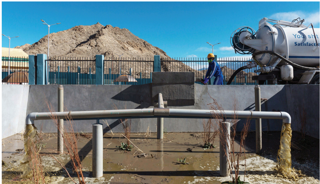
Blue Water Company staff discharges fecal sludge onto the drying bed (photo by BORDA).
