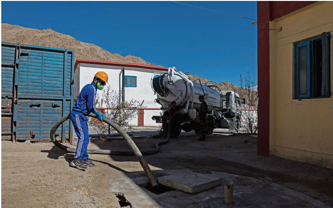
Blue Water Company (BWC) staff cleans a septic tank at army facility (photo by BWC).
