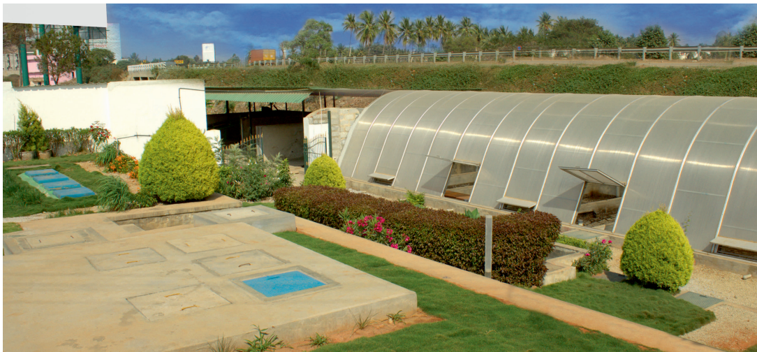
India's first fecal sludge treatment plant in Devanahalli, Karnataka (photo by CDD Society/BORDA).
