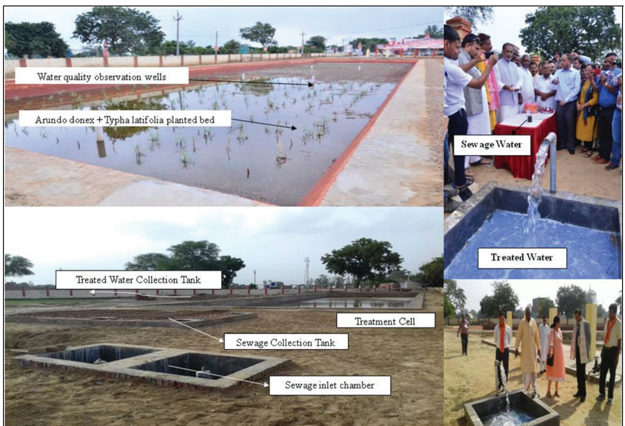
Figure 36:Layout of Pilot Rural Household Sewage Water Treatment System
