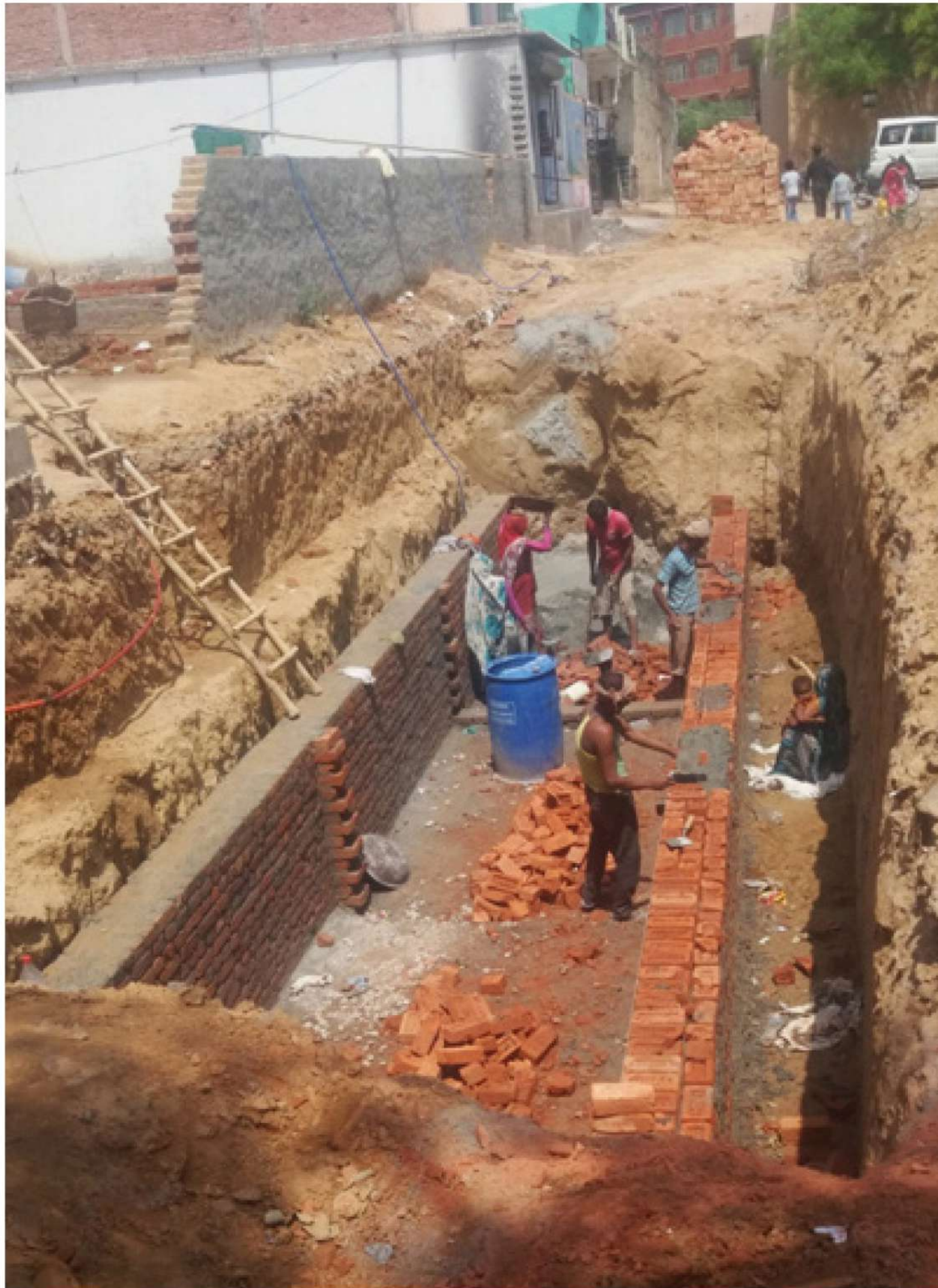
CONSTRUCTION OF RAFT FOR PLACEMENT OF BIO DIGESTER BELOW THE STREET
