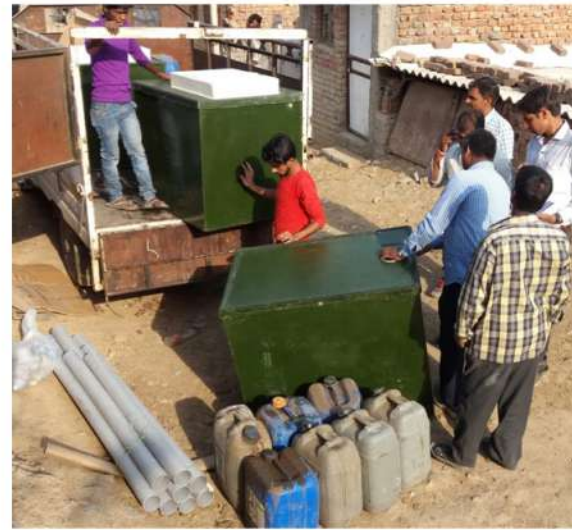
Bio digester being unloaded on site
