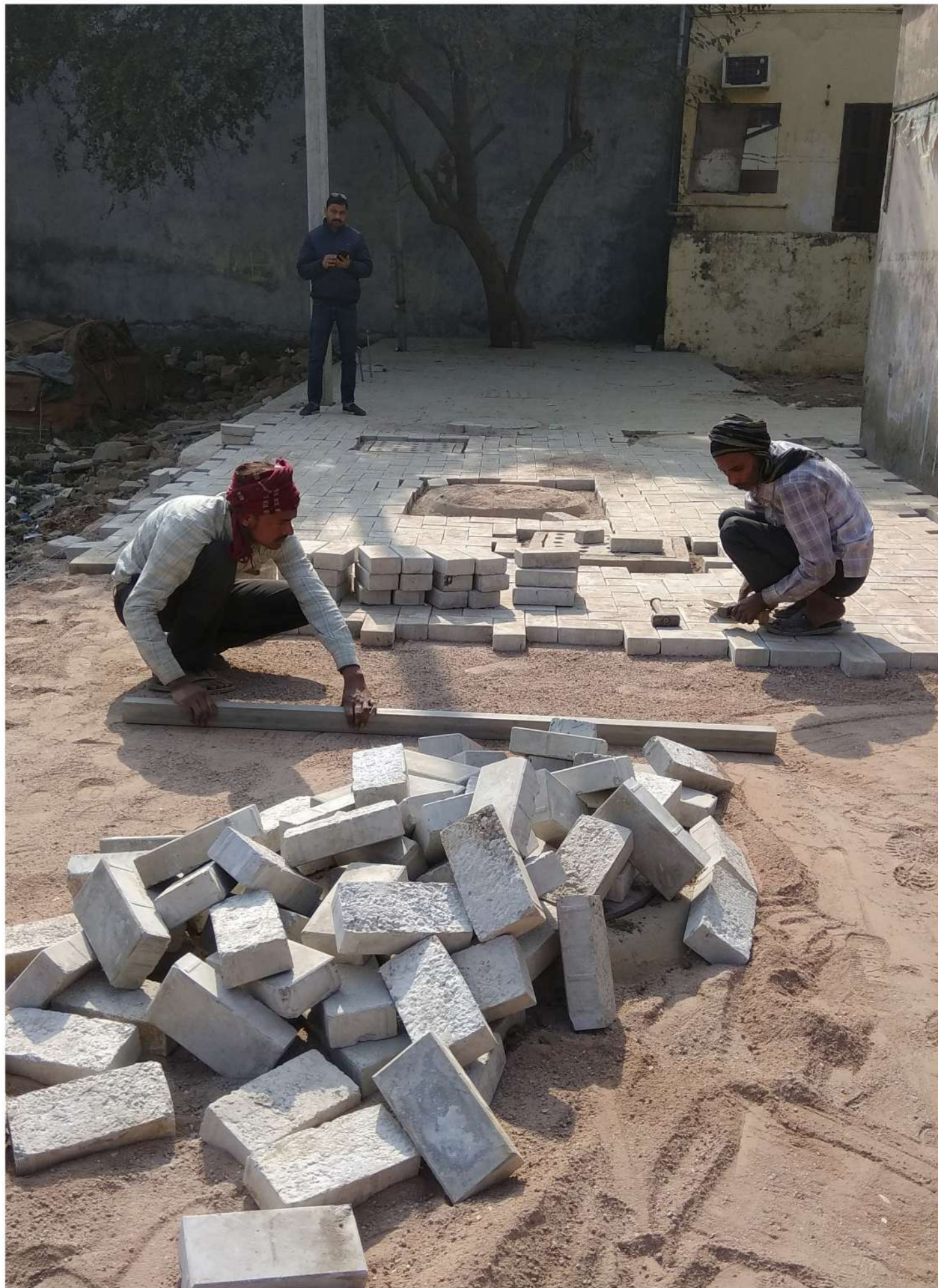
RESURFACING THE STREET
