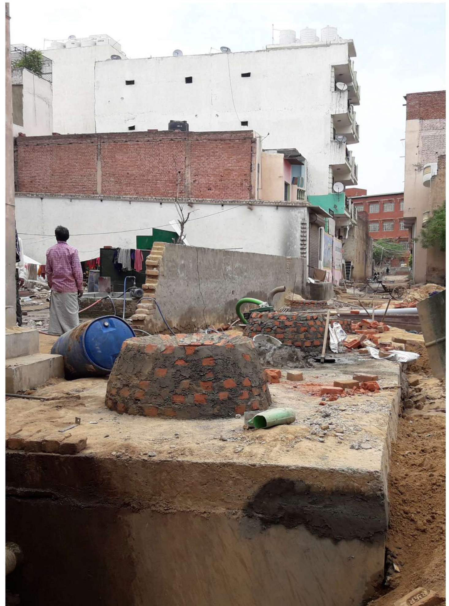
PLUMBING WORK BELOW THE STREET SURFACE
