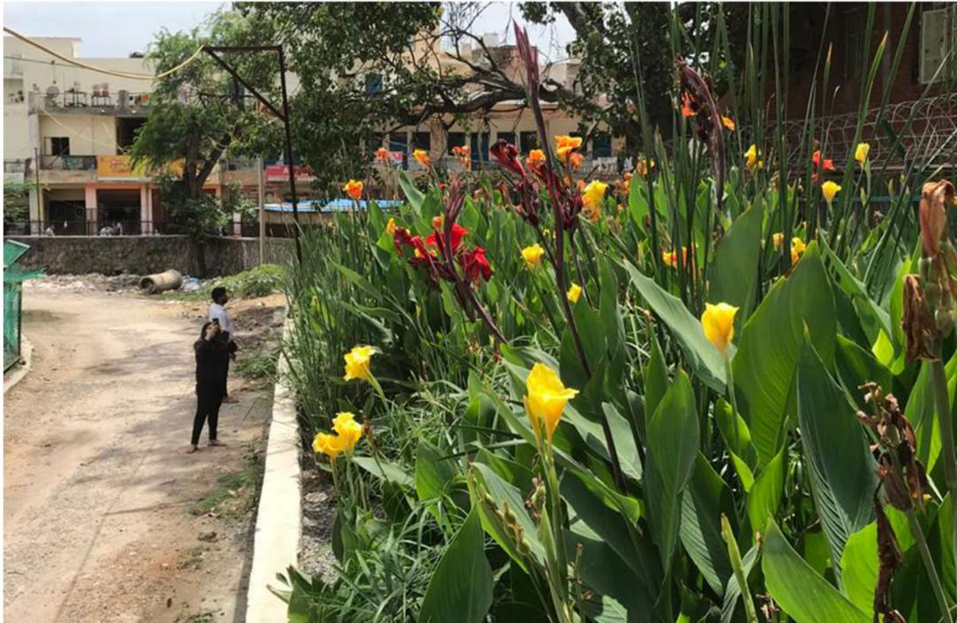
Root-zone treatment in the constructed Wetland
