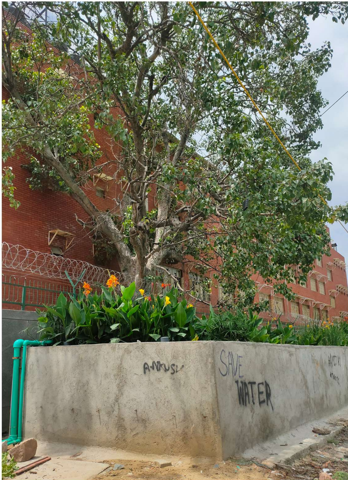
CONSTRUCTED WETLAND (REED BED) ADJOINING THE JOHAR
