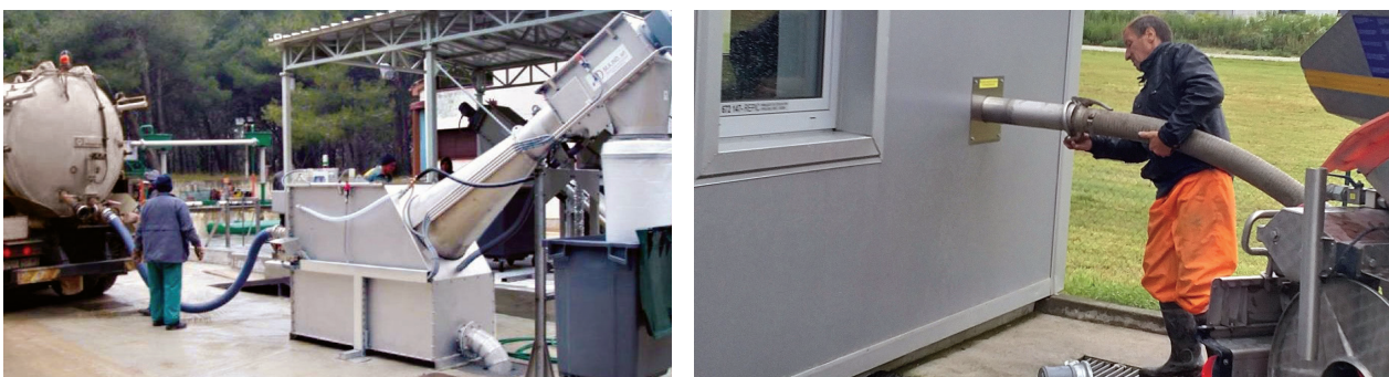
Figure 64: Typical photographs of the septage receiving station
