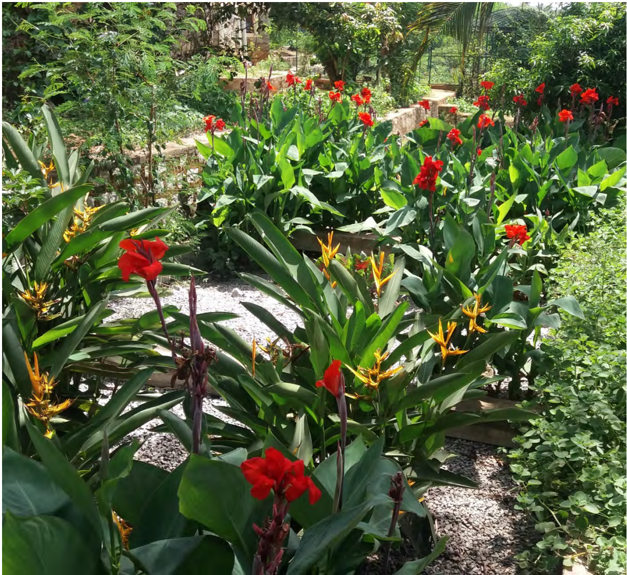
Figure 64: Planted gravel filter for wastewater polishing (Photo: Milan Basil Kurian).
