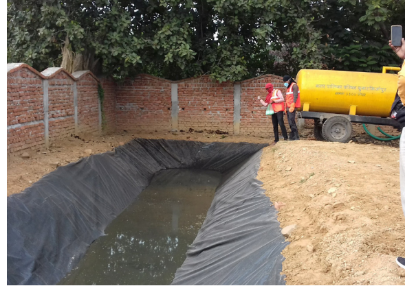
Trenching site for temporary FS disposal in Chunar
