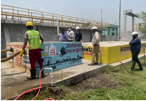
Bijnor co-treatment plant (20 KLD), commissioned in July 2022
